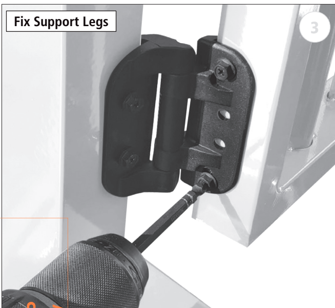
3. For hinges with support legs also fix to post.
