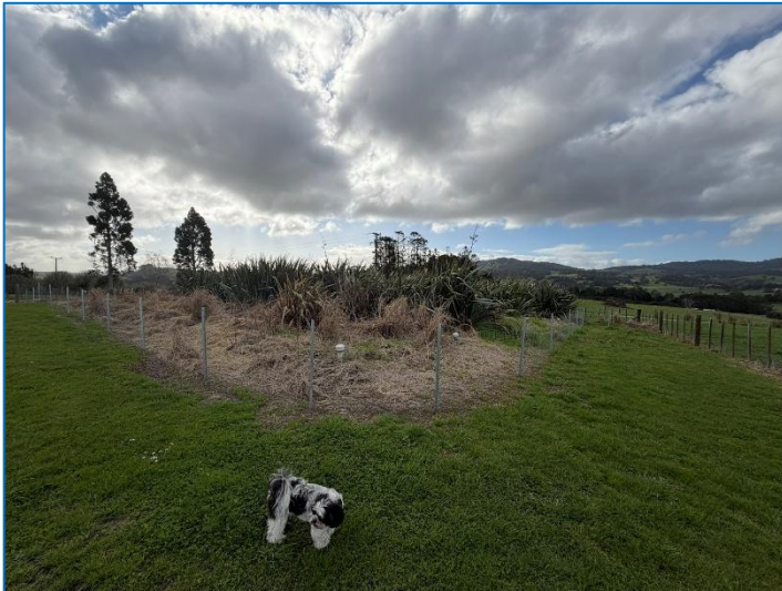
Photograph 2: Mounded evapotranspiration beds for onsite wastewater disposal.
