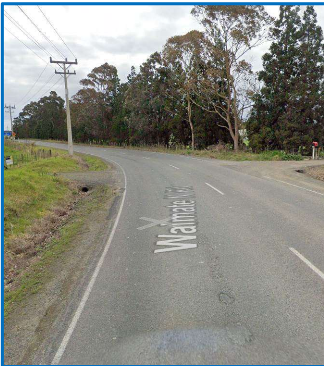
Before – Note edge line position.
