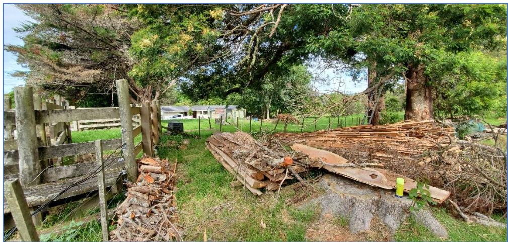
Figure 3 – view of rear boundary and neighbour's house to the east
