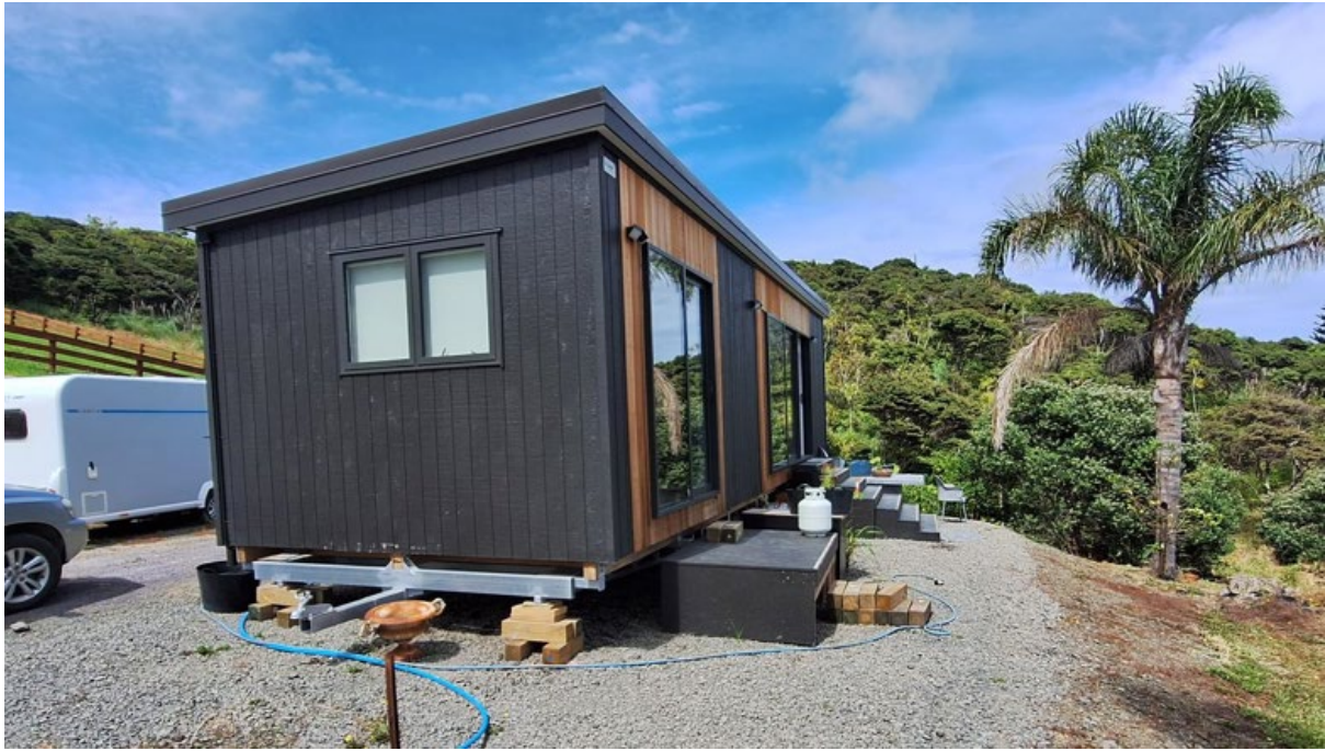
Figure 3 – Existing Transportable home
