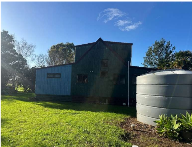
Figure 7- 1 x 25000L water tank. Proposed Lot 1, Dwelling 1
