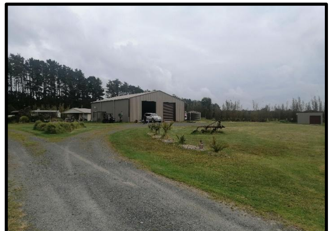
Figure 8: Existing shed, and ancillary buildings to be contained within Proposed Lot 2. Consented under RC2170177.
