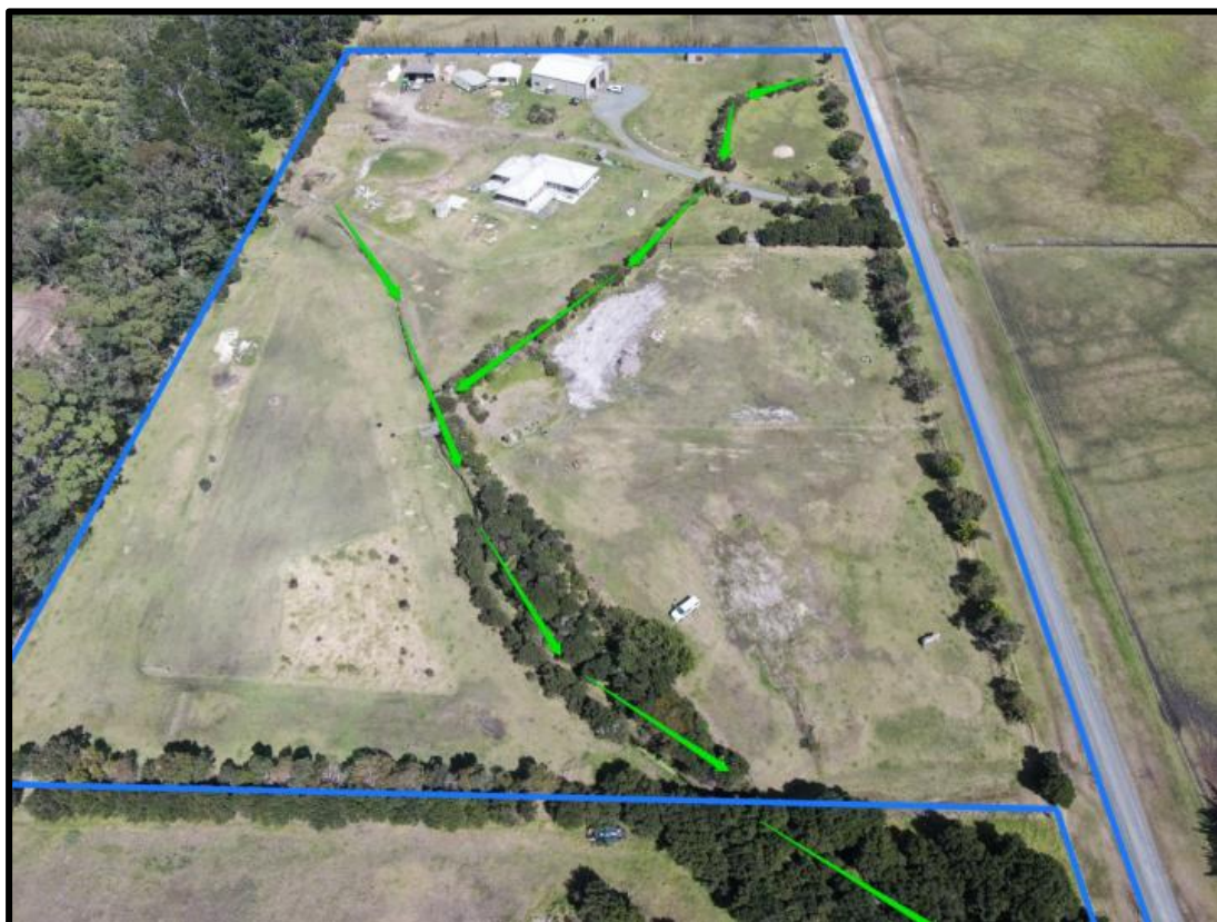
Figure 5: Aerial image of the site showing site boundaries in blue and existing overland flow path channel in green (taken from WJ Report). Proposed Lot 1 is located where white vehicle can be seen in the lower right corner of the image.
