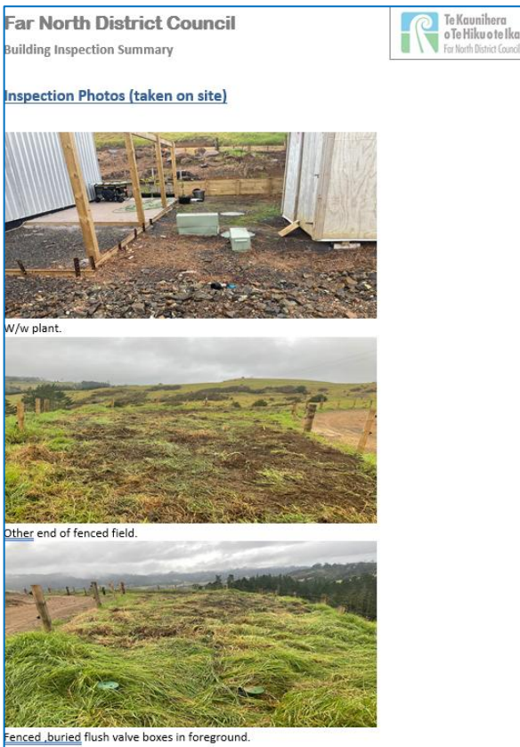
Figure 2: Inspection Photographs EBC-2022-729-0 (Sourced from Far North District Property File Records).
