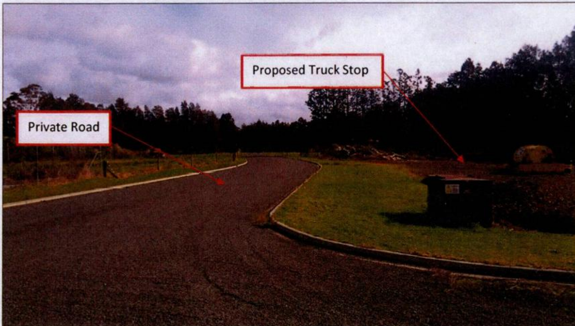
Figure 4: Private Road in the vicinity of the site
