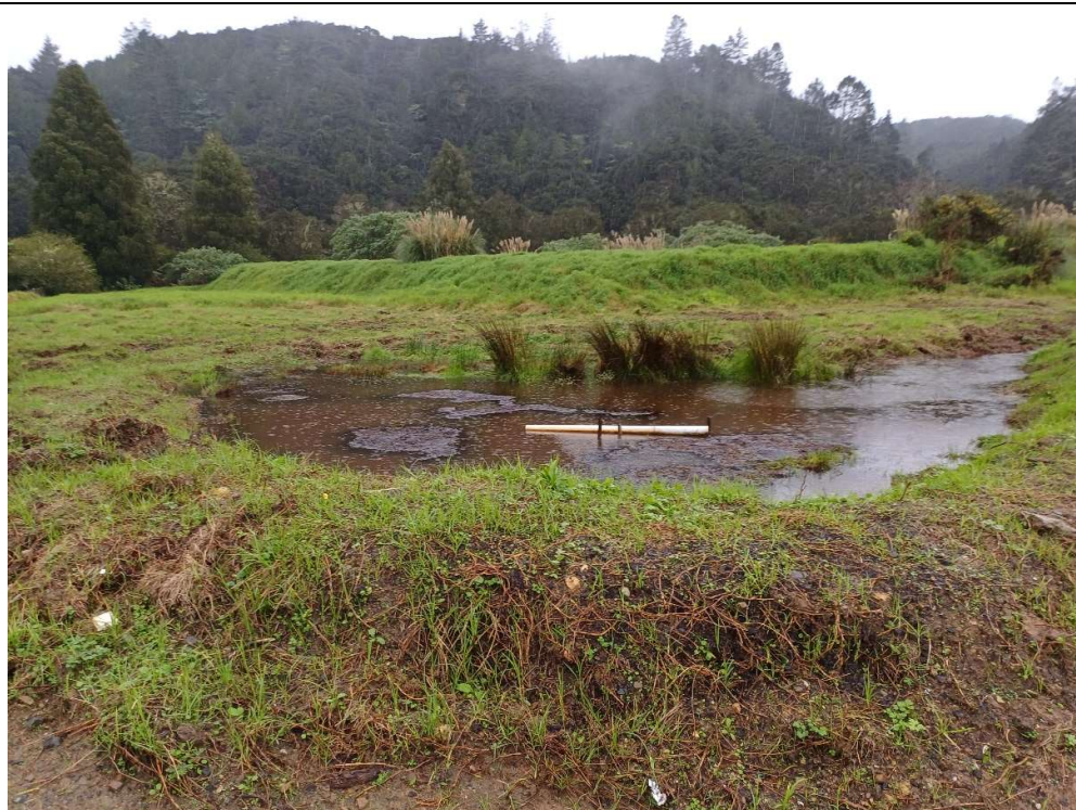
3. Leachate disposal spreader bar
