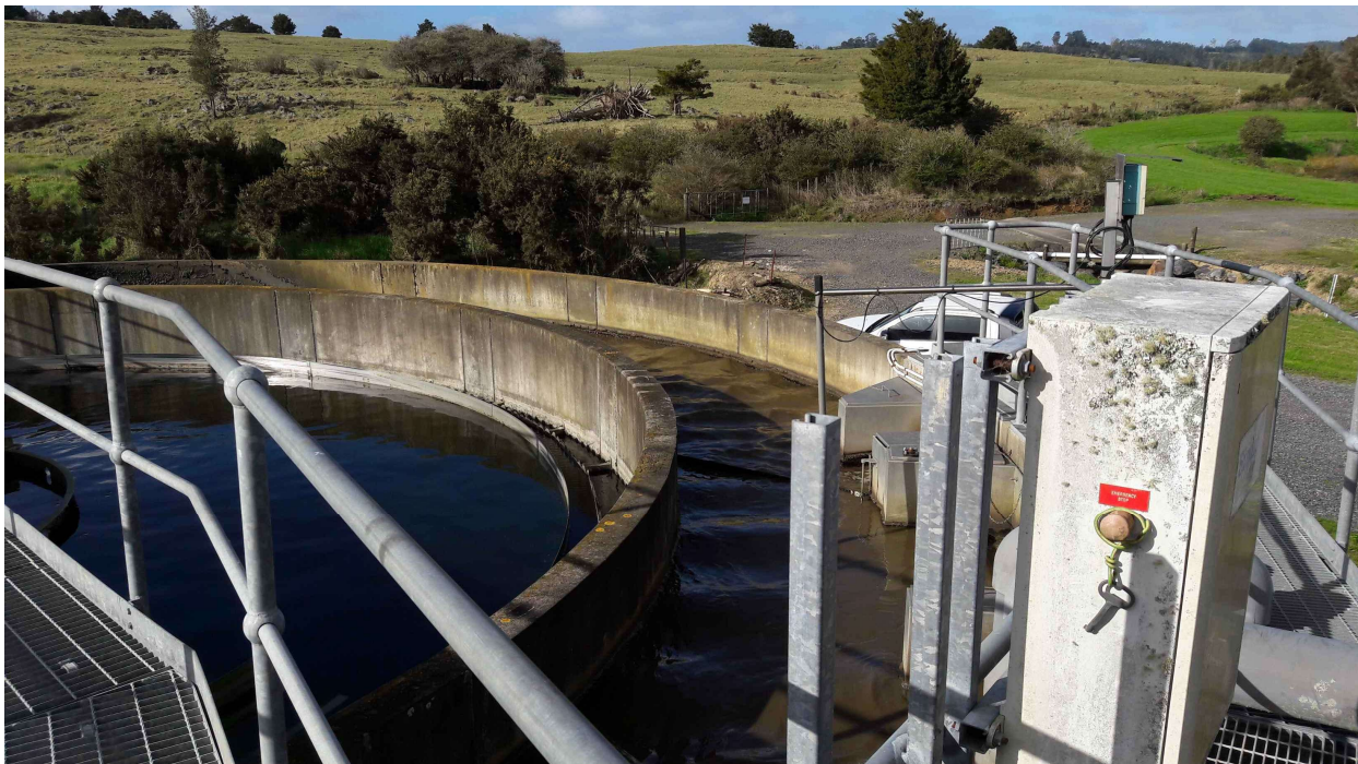
Photo - Kawakawa WWTP view of proposed earthworks site from the bioreactor tank
