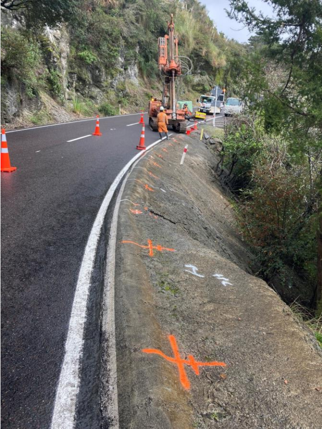
HRRi Mangamuka Rd Guardrail Installation
