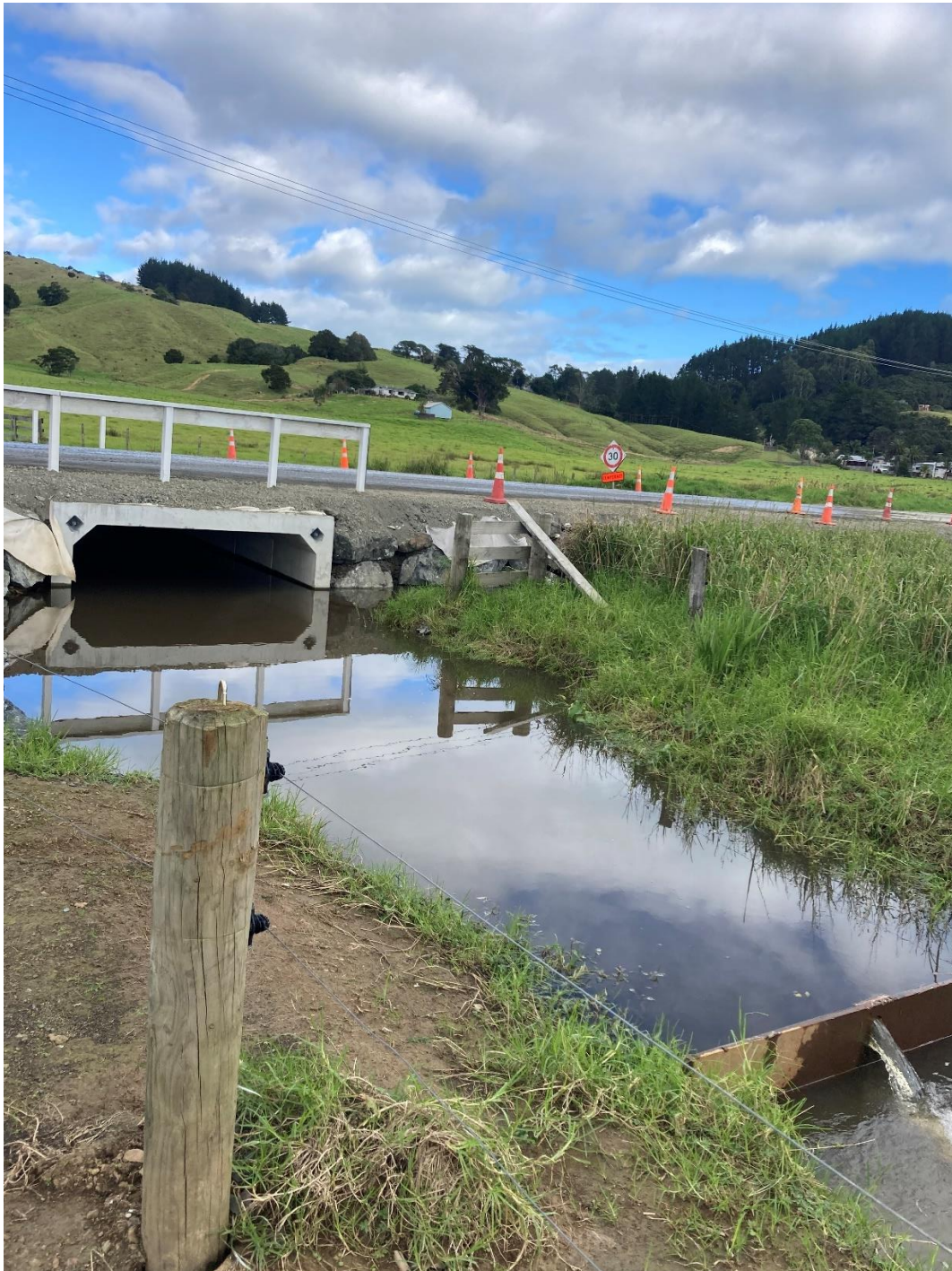
Kaitaia Awaroa Rd Box Cuvlert Replacement
