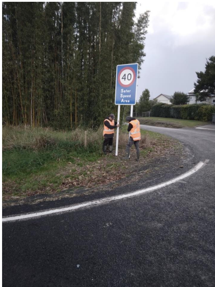
New Speed Management Signs Installed
