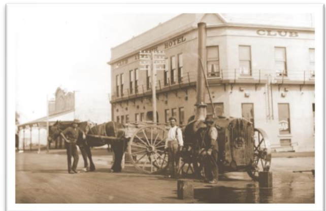
Horse drawn bitumen sprayer ready for sealing the main street of Opunake (right side photo)
