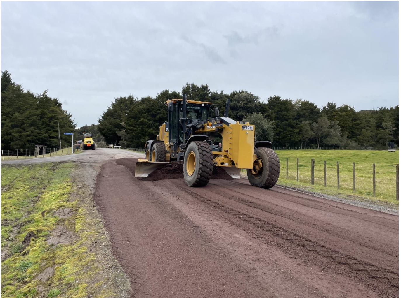
Ngawhitu Rd unsealed overlay – Brian in action.
