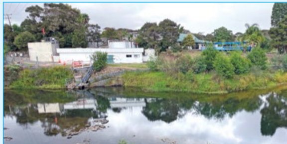
Repairs to the riverbank at the Paihia WTP will start soon.
