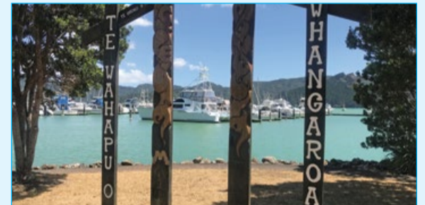
A section of the main road into Whangaroa is reduced to one lane.
