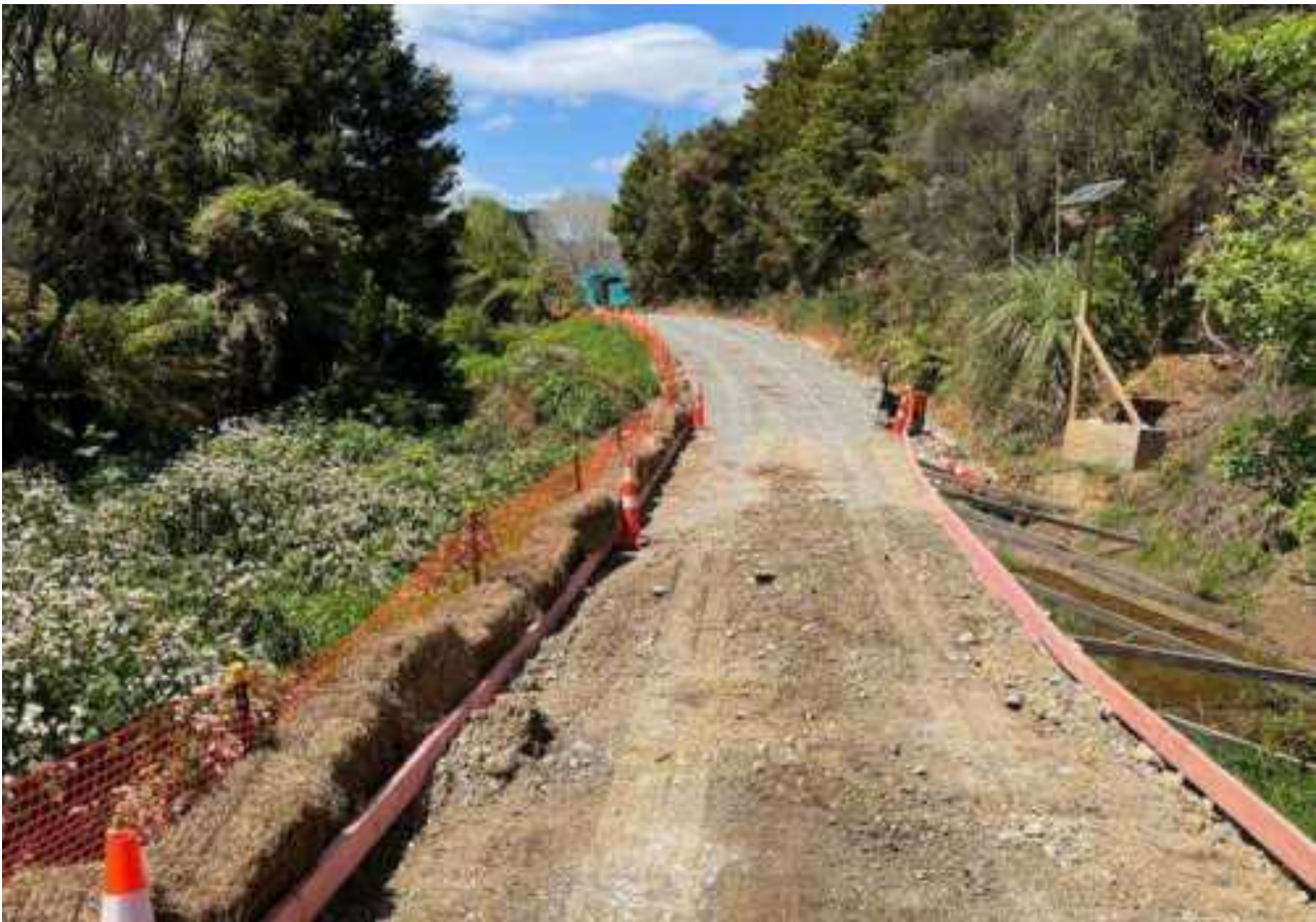
Figure 5: Photograph of culvert crossing being upgraded to concrete finish
