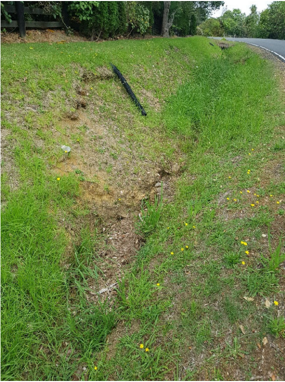
Roadside drain outside 80A Pa Rd – looking South-west
