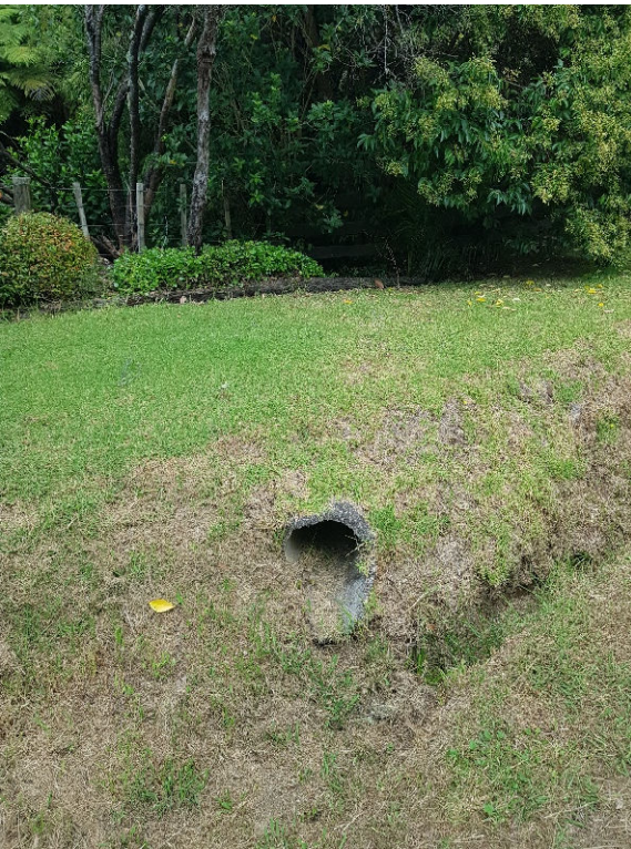
450mm culvert from open drain into Pa Rd swale
