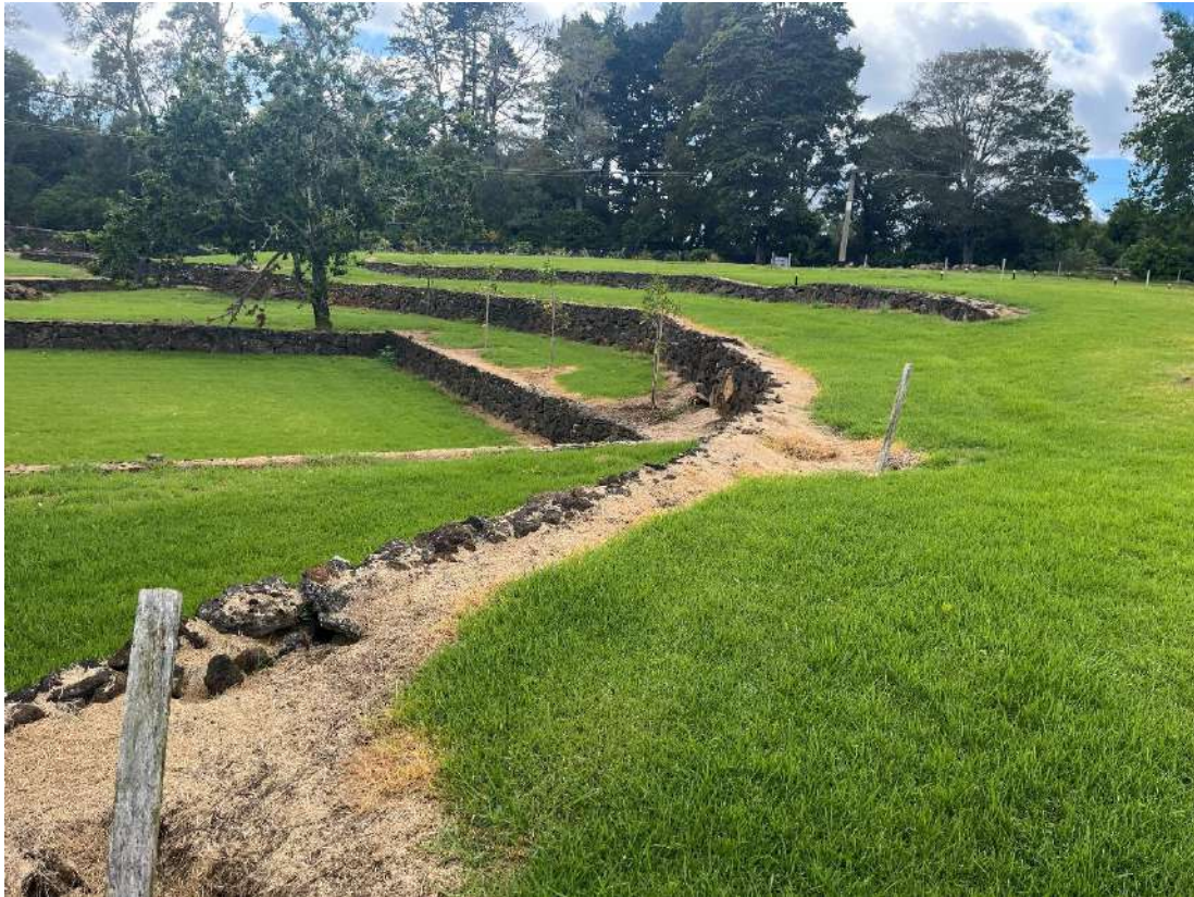
Photograph 1: Terracing formed by excavation, filling, rock wall construction (“landscape contouring”, c2003, FNDC RC 2030517).
