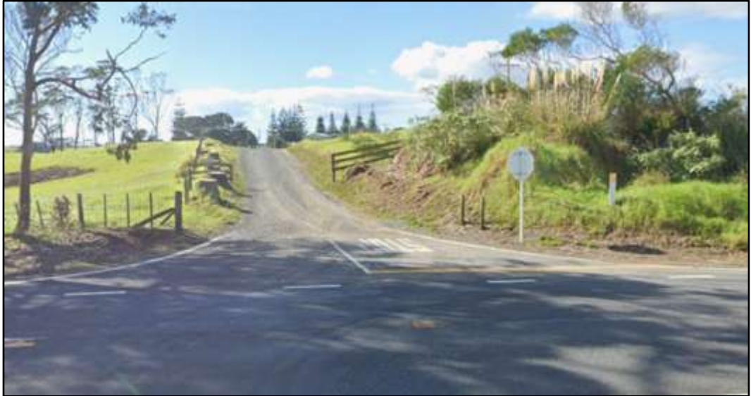
Figure 2: SH1/Srhoj Road intersection
