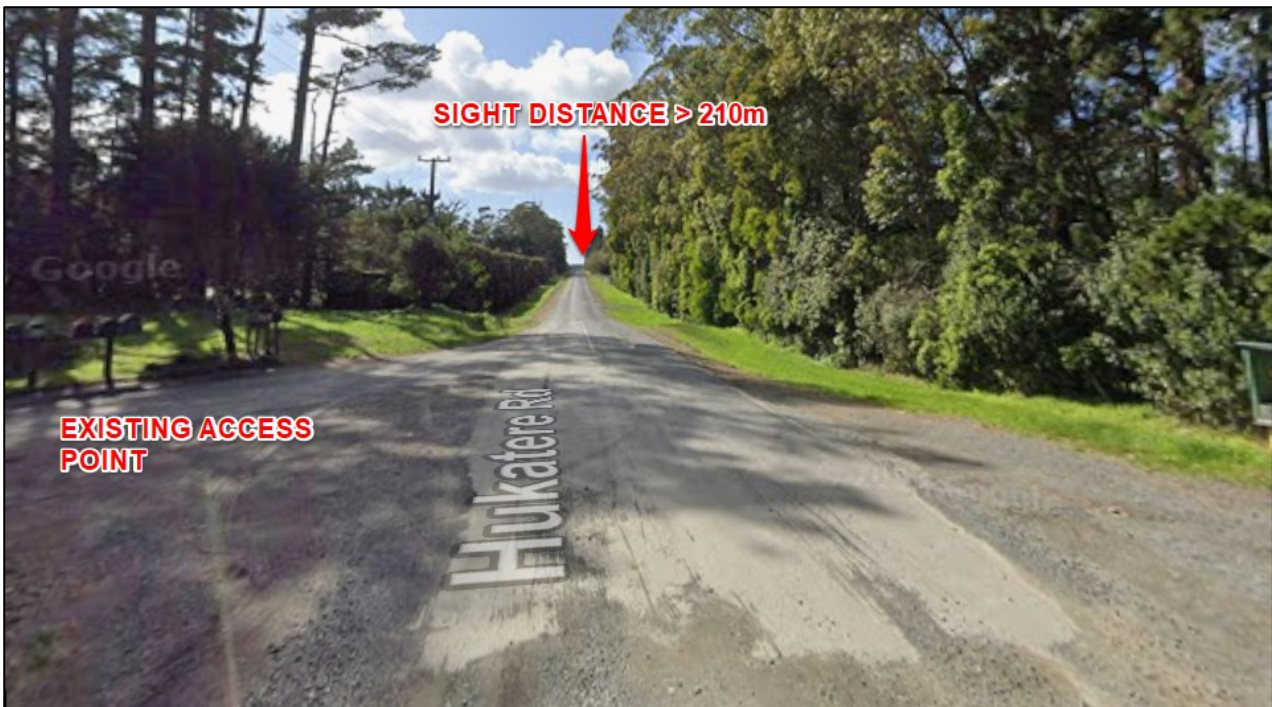
Figure 6: Annotated photo showing available sight distance to the northeast
