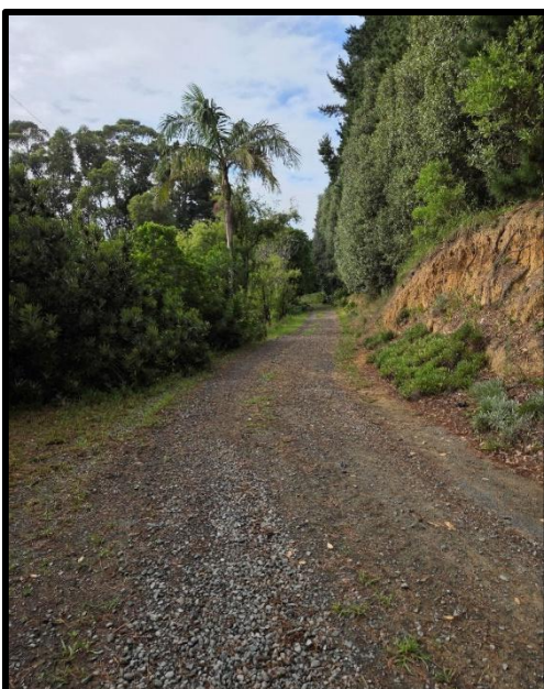
Figure 8: Internal access leg to the subject site.
