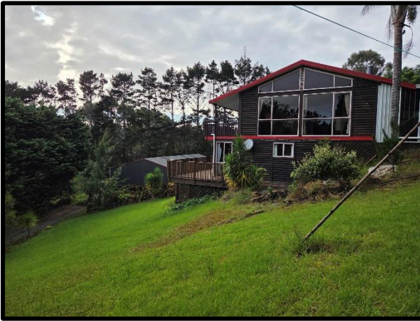
Figure 4: Image of the existing dwelling and shed. Taken from the northern area of Lot 1.
