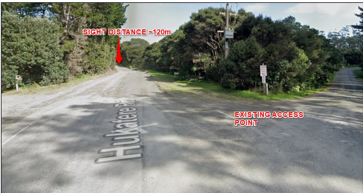
Figure 7: Annotated photo showing available sight distance to the southwest
