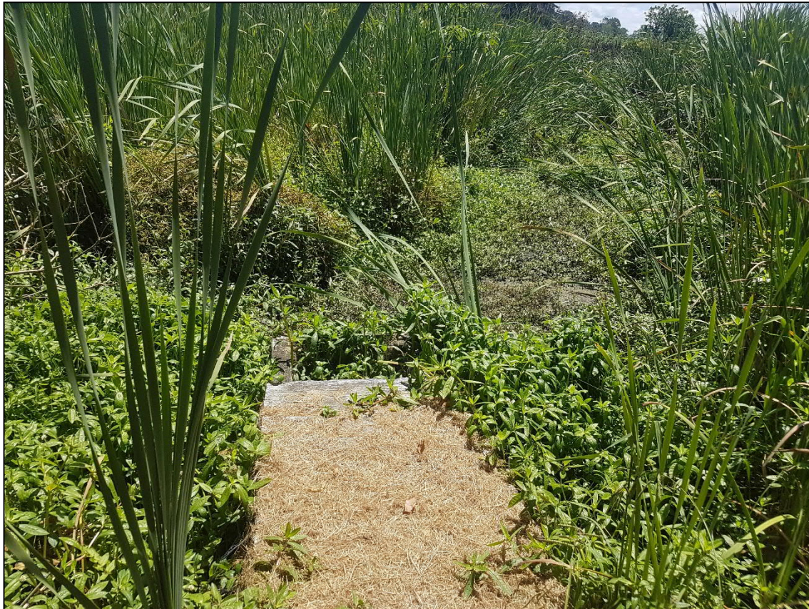
Figure 3-3: View of Kohukohu WWTP Constructed Wetland
