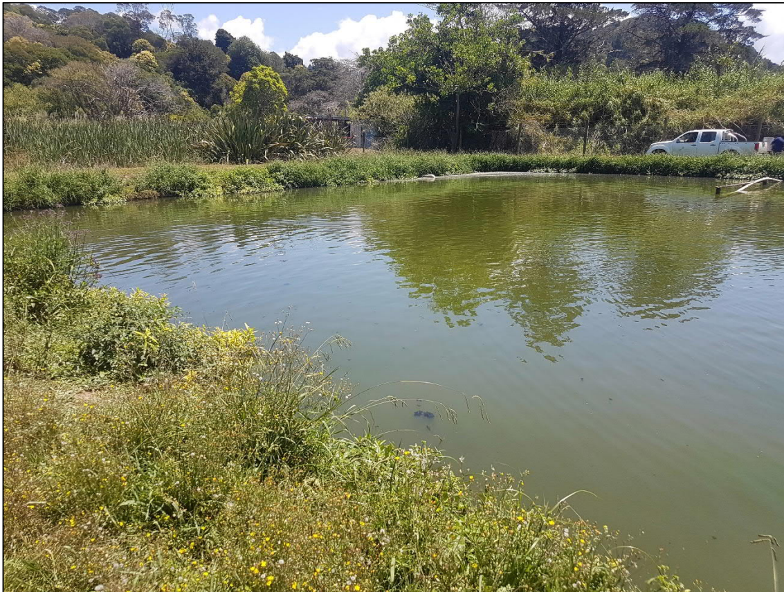
Figure 3-2: Kohukohu WWTP Oxidation Pond
