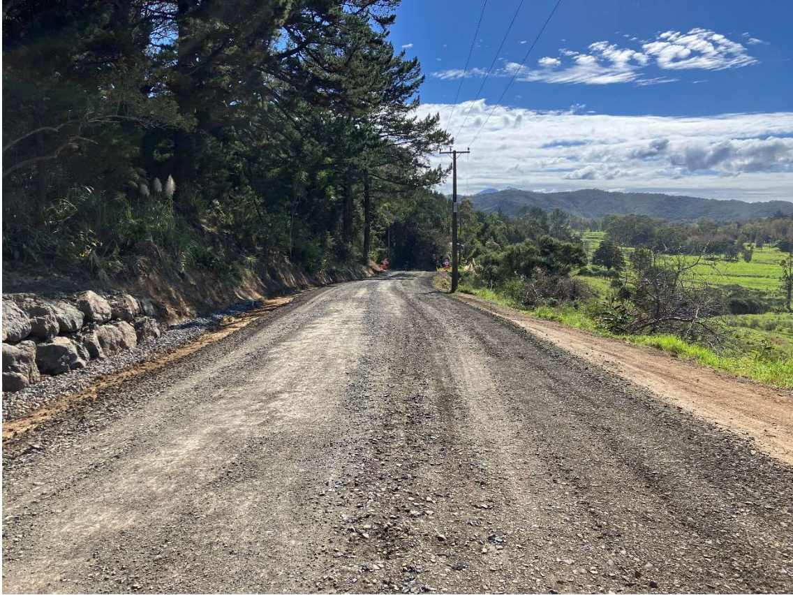
Pawarenga Road Seal Extension
