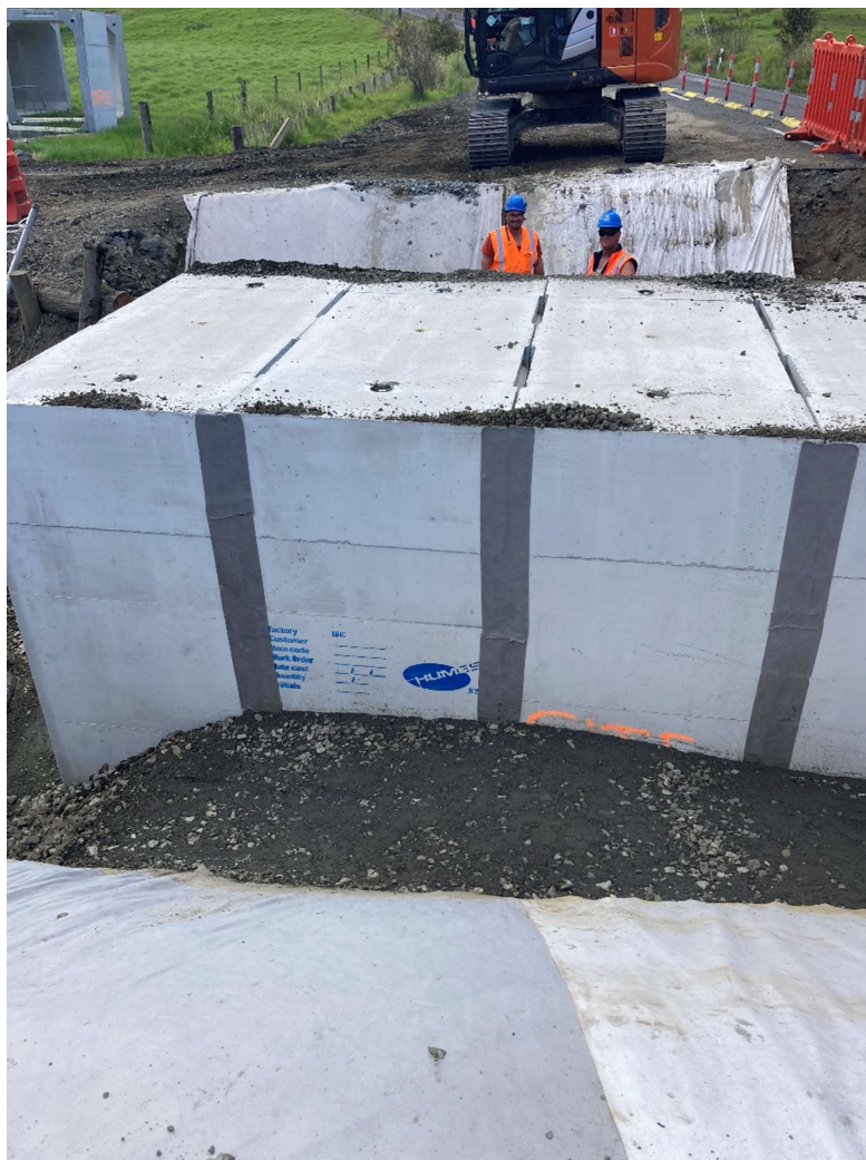
Kaitaia Awaroa Rd Box Culvert Installation
