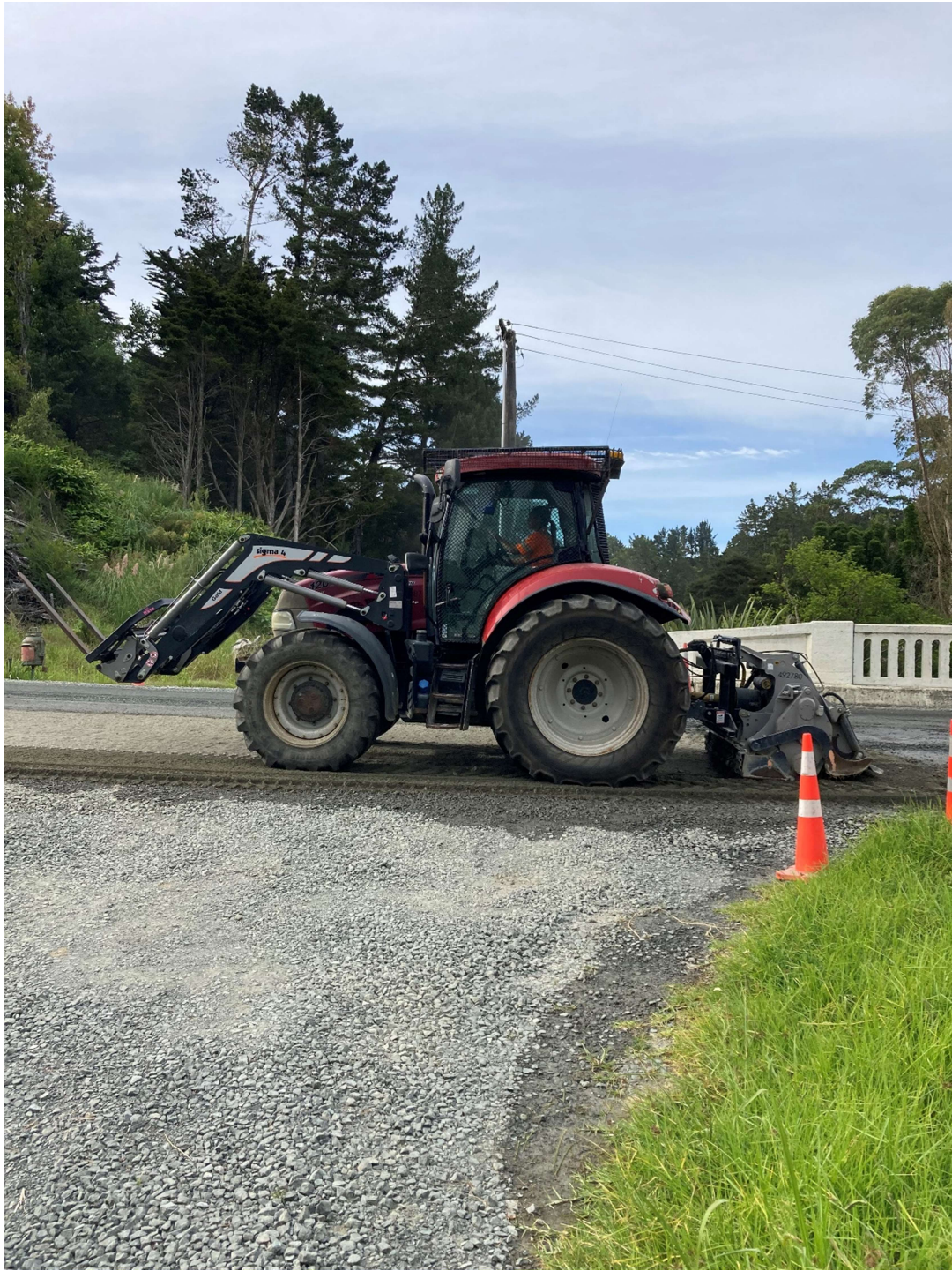
Peria Road Seal Extension Slip Repair Pavement Completion
