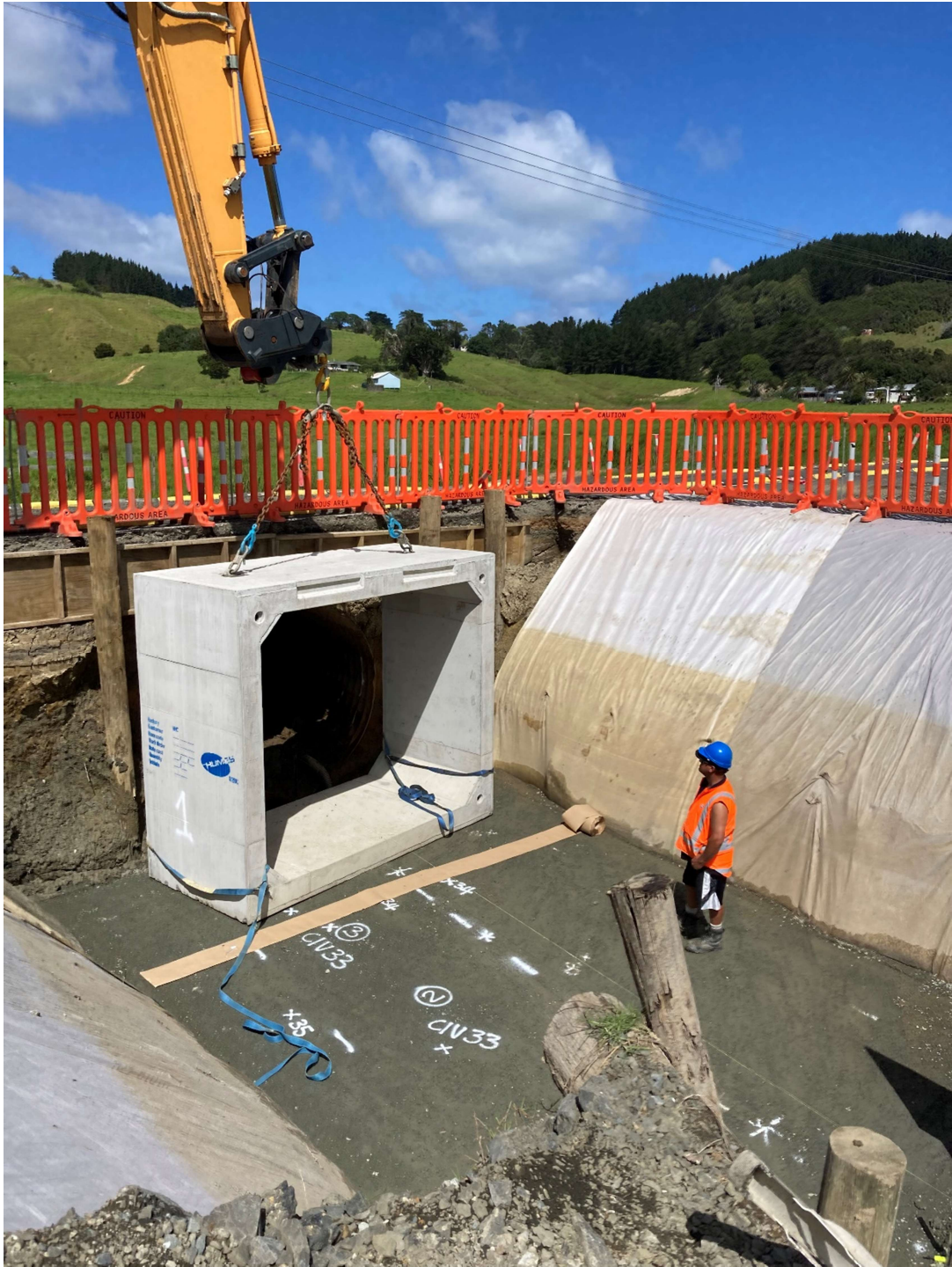
Kaitaia Awaroa Rd Box Culvert Installation
