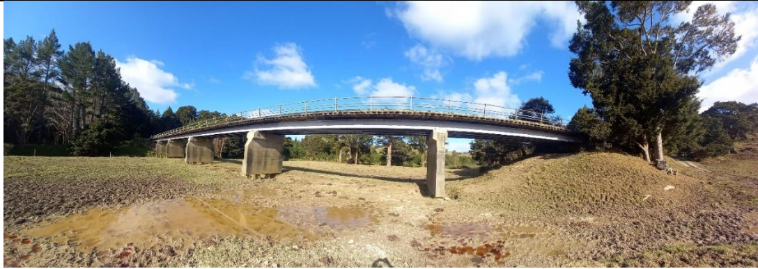
Ararua Bridge No. 168 – structural beam painting works
