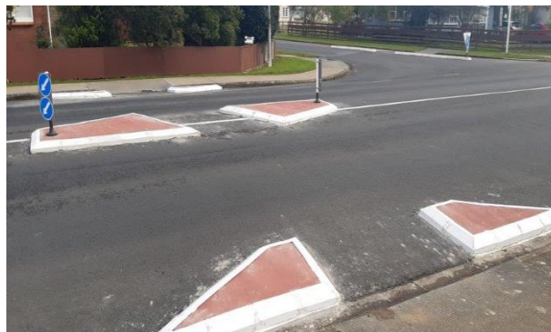
Pukepoto Rd/Lake Rd Intersection
