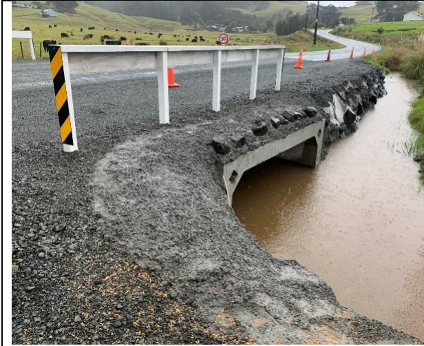
Kaitaia-Awaroa D41 Culvert Replacement
