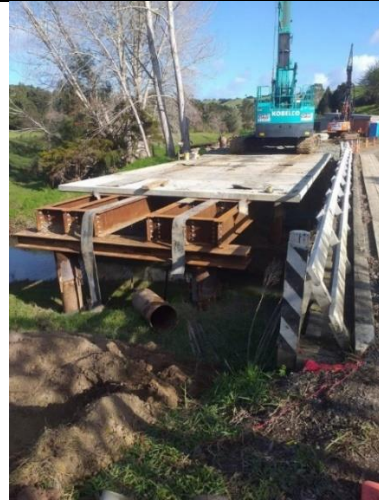
Churtons Road Bridge C13 Replacement – ongoing construction of temporary crossing
