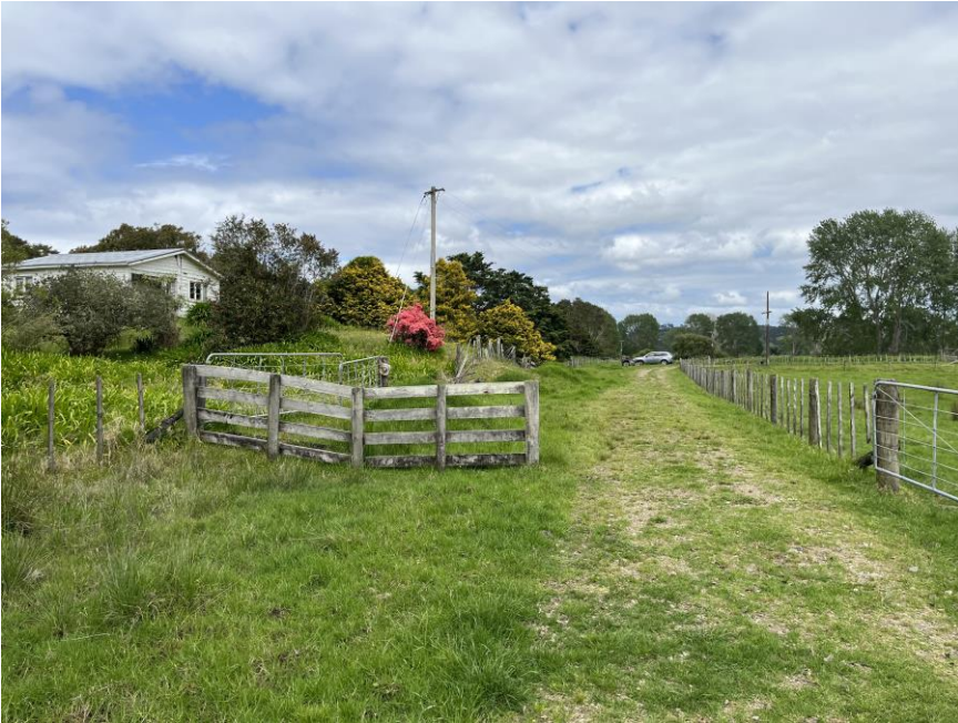
Photograph 6: Access over easement C (Final Scheme Plan), showing formation within stopped road. Note that the overhead power lines to the left of the photo are now redundant, as underground power has been supplied from a transformer at the base of the power pole to the right.
