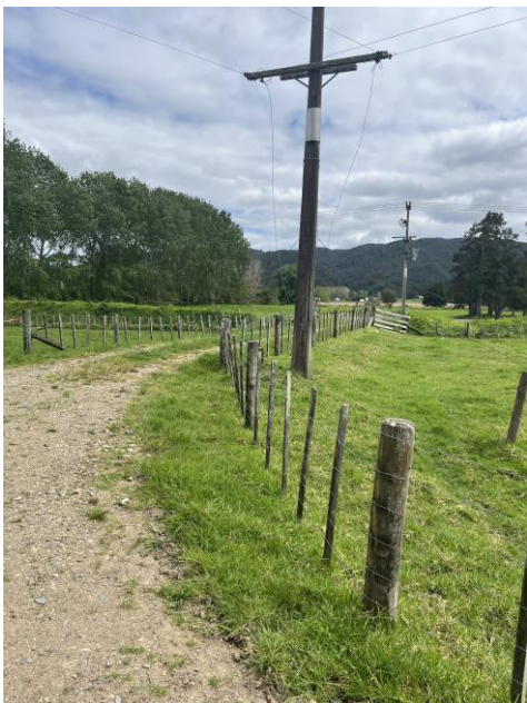
Photograph 5: Formed access over easements A and B (Final Scheme). Looking back towards State Highway 1.
