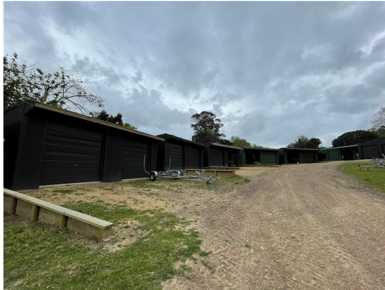
Figure 4: Existing sheds that are the same design as the proposed shed. Refer to Appendix 2 for full set of shed plans. Photo taken 18/10/2023.
