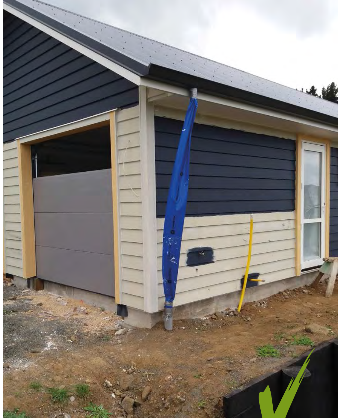
Temporary drainpipe installed on house under construction.
