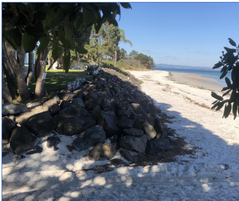
Figure 4: Existing hard protection structure
