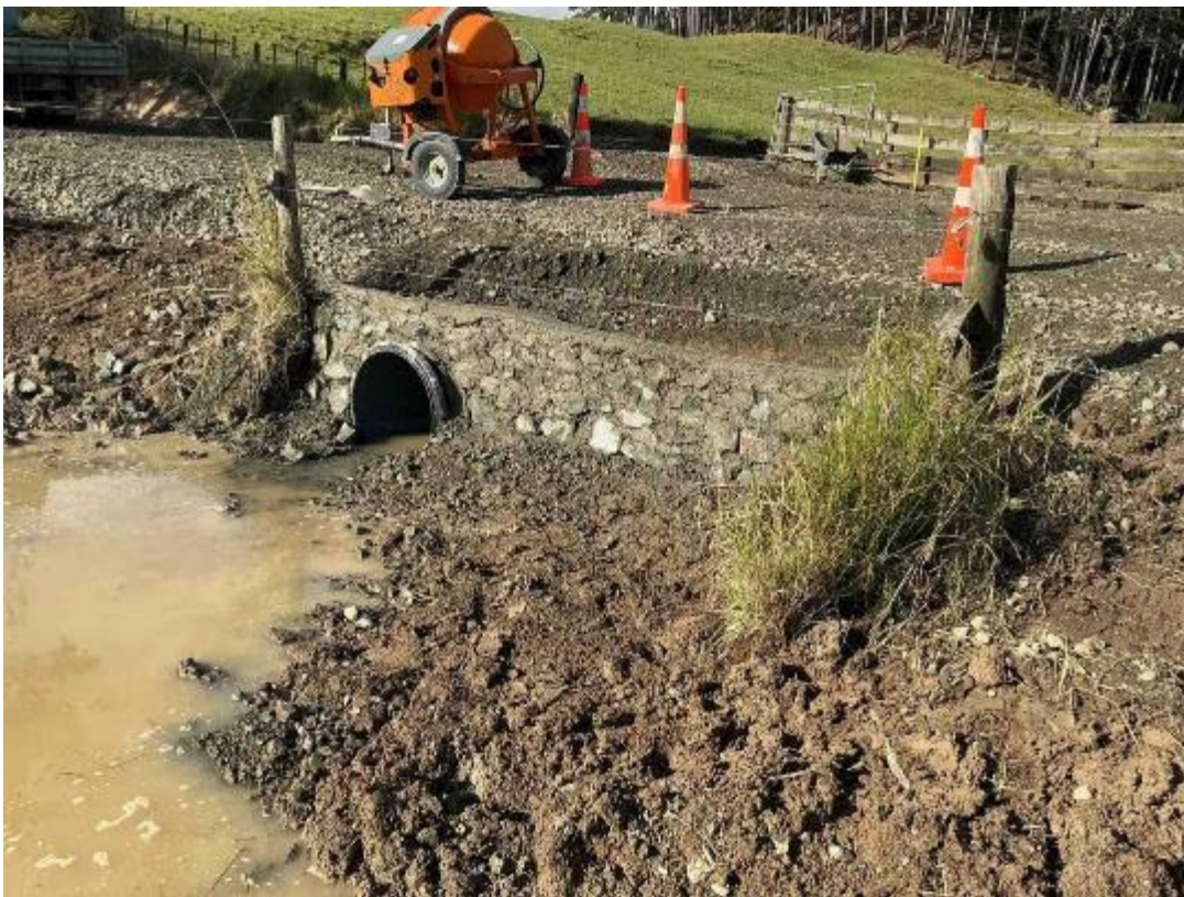
Peria Valley Rd, Kaitaia – Culvert Headwall
