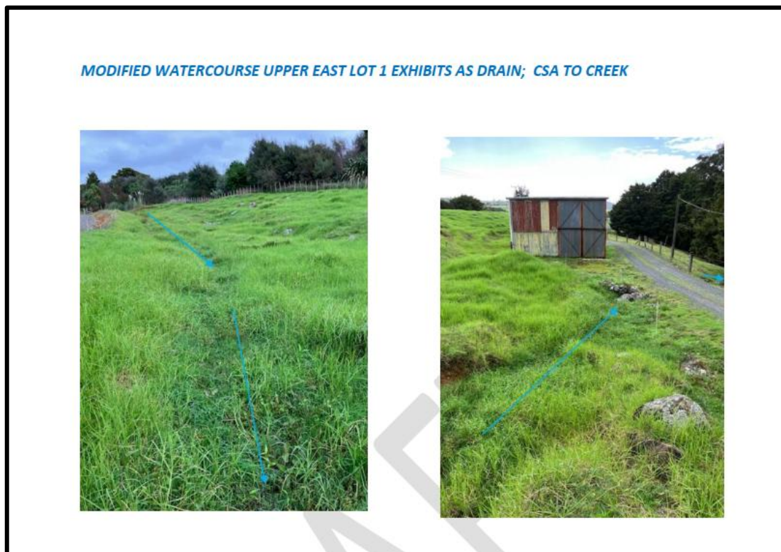
Figure 26: Image of modified watercourse where culvert will be placed under new accessway within Easement C. The existing culvert under the existing accessway is shown in the image to the right.
