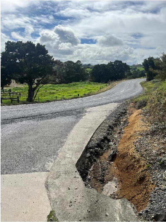
Existing open drain to be rock lined.
