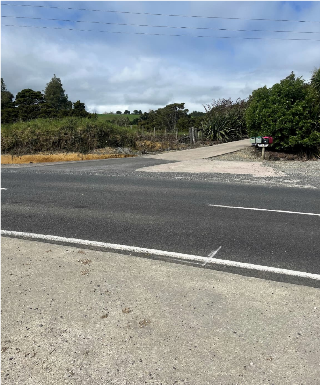
View of existing vehicle crossing for Lot 1, DP 516974, Lots 1 and 2, DP 566354 and access to the ROW serving the new proposed lot 2 on the left.
