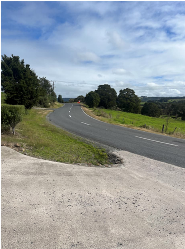
Vehicle crossing sight distance towards the South.
