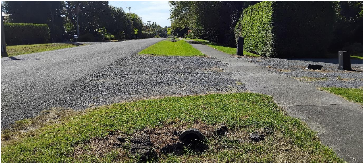
Figure 6: Existing Culvert from Kendall Road towards property.
