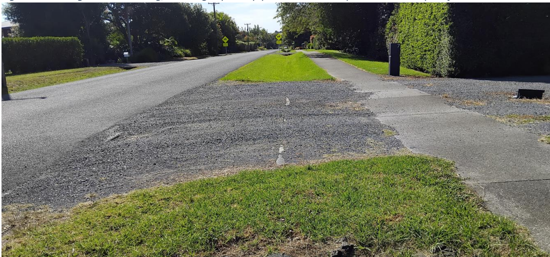
Figure 1: Existing vehicle crossing, showing exposed pipe culvert and dispersed stone chip surface
