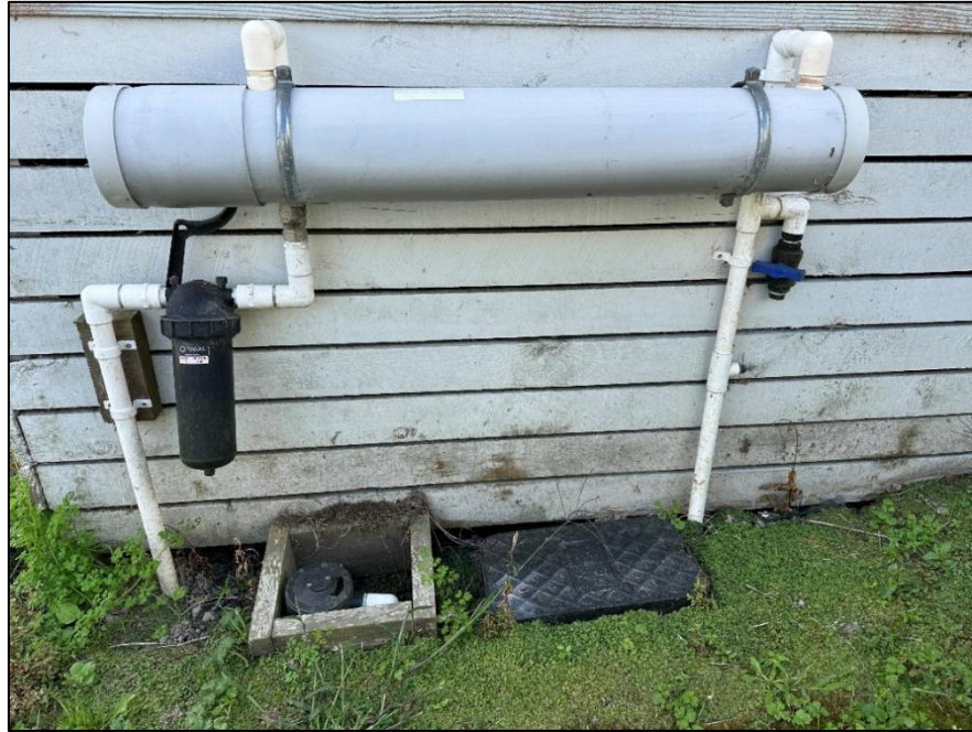
Figure 4. The UV unit and sequencing valve
