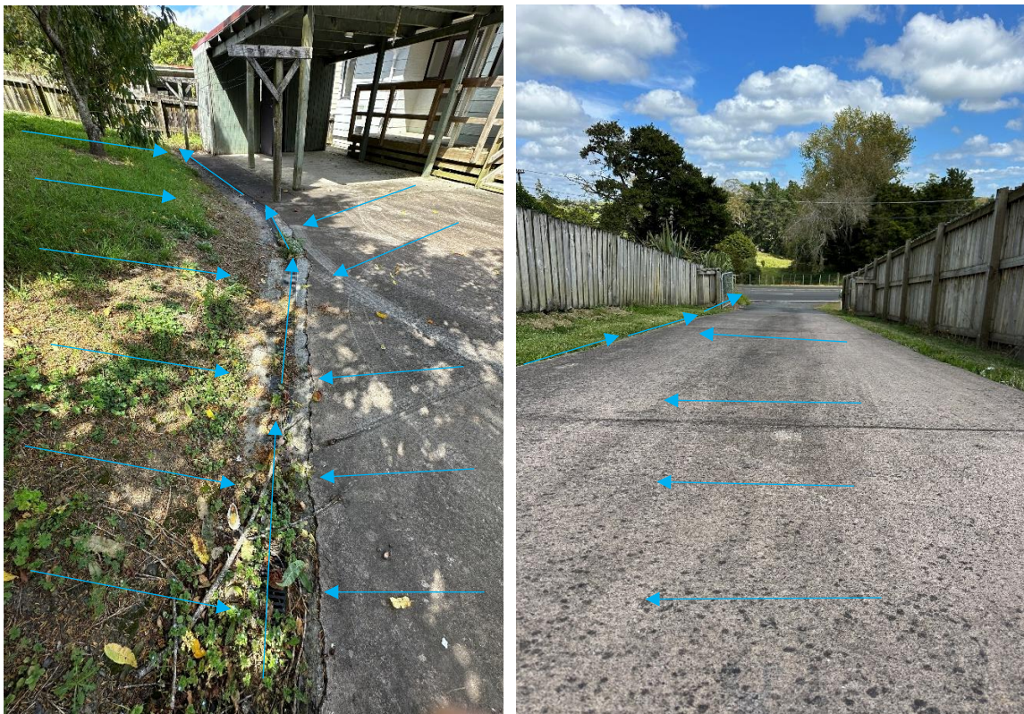
Figure 8. Driveway Stormwater Flow Direction Blue arrows indicate surface water flow paths
