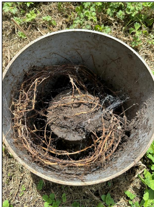
Figure 12. Sequencing Valve Root Intrusion
