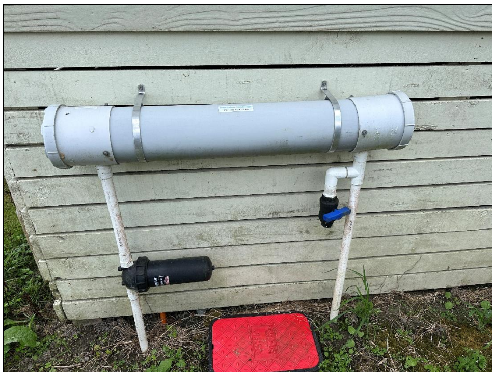
Figure 10. The UV unit and mesh filter
