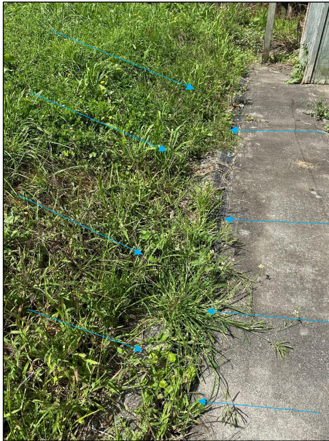
Figure 16. Channel Drain and Driveway near garage grading Blue arrows indicate surface water flow paths
