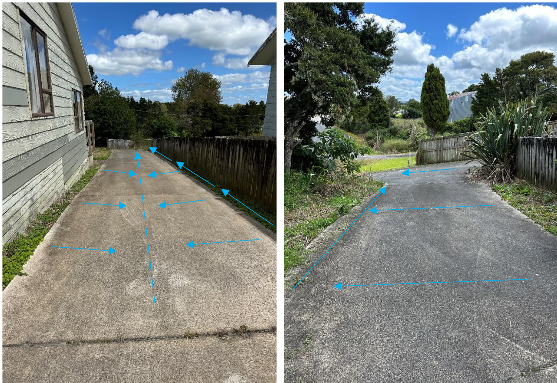
Figure 15. Driveway Stormwater Flow Direction Blue arrows indicate surface water flow paths
