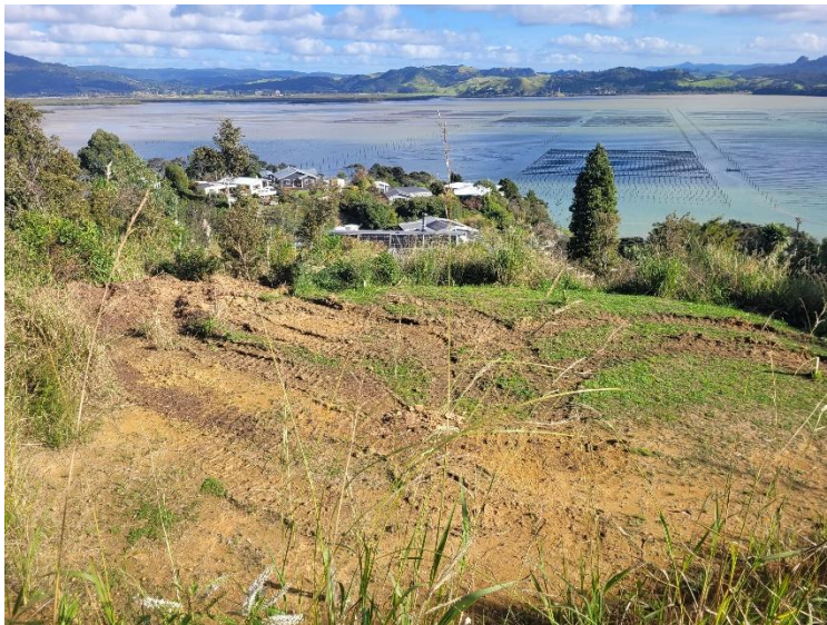
Photo provided by applicant. DMRU building site, looking southwest.
