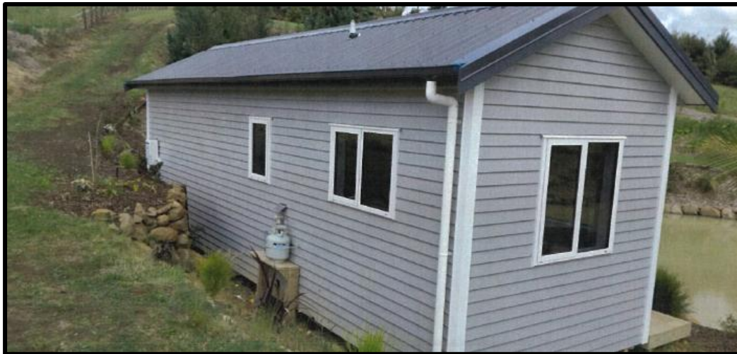
Figure 7: Southern side of cabin where setback infringement occurs.
