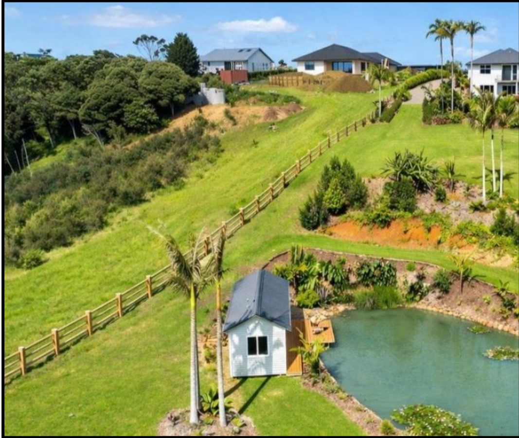
Figure 6: Image showing location of subject cabin and adjoining Lot 43 DP 532487 where setback infringement occurs.
