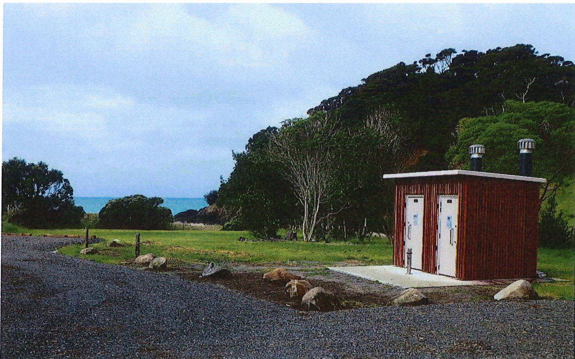
Photo 4. The new sealed-vault Permaloo toilets are unobtrusive and are working well.
