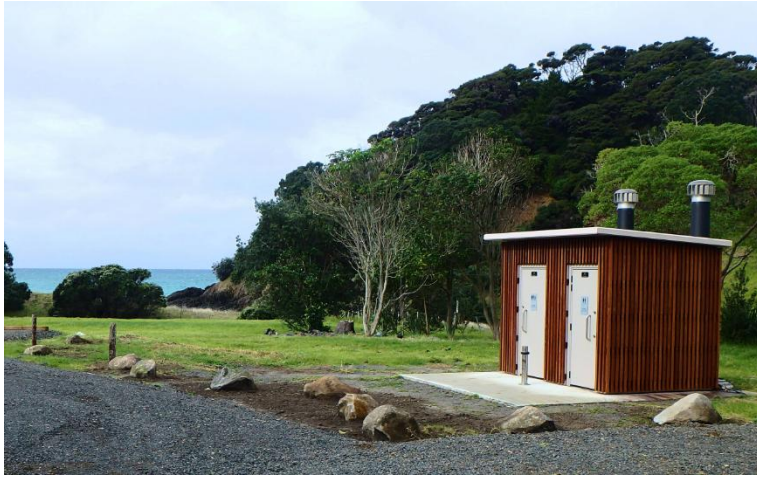
Photograph of new toilet facilities recently constructed by the public carpark on the site.
