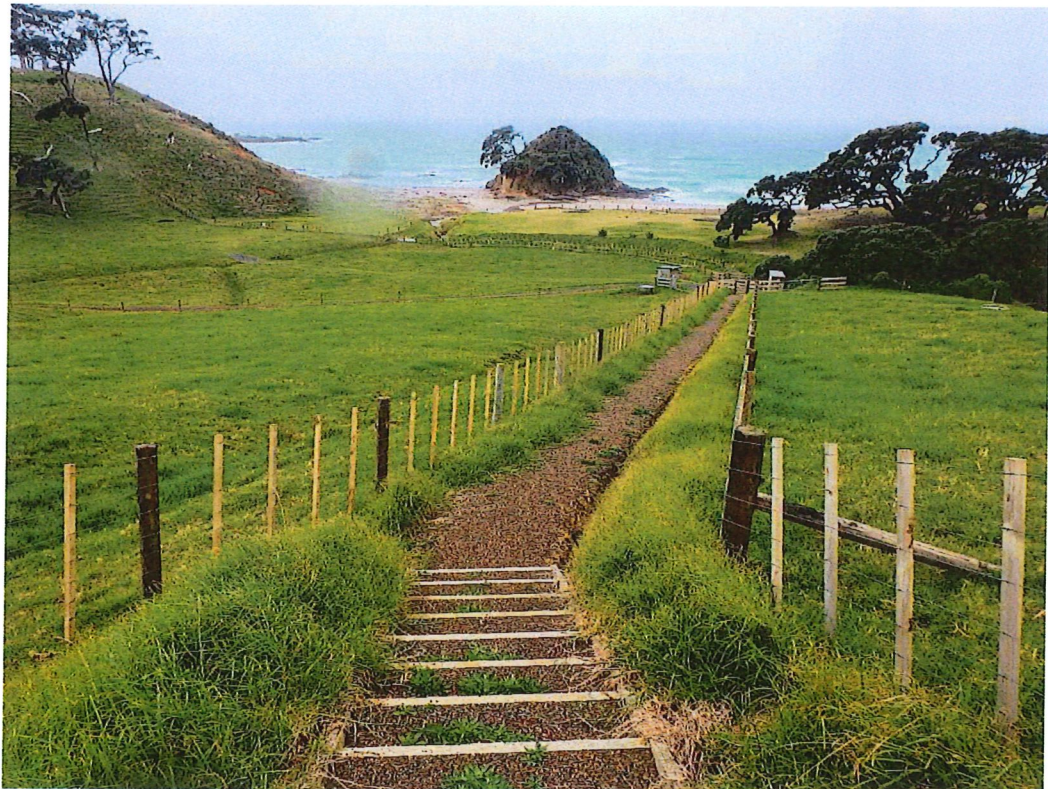
Photo 8. View of new toilet location approaching on walkway down from viewing area.
