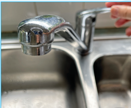
The Kerikeri-Waipapa water network has undergone additional work to flush out manganese.
