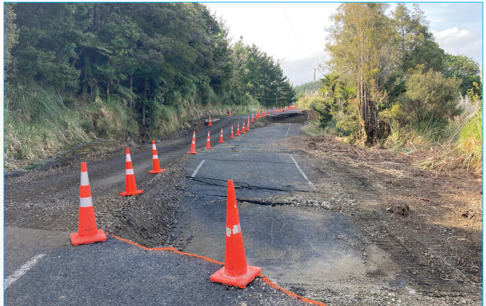
Repairs to two major slips on West Coast Road are expected to start early this year but may take some time. A detour remains in place for heavy vehicles at the Kohukohu slip.
