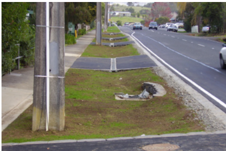
Fig.3 Henderson Valley Road – newly constructed road side swales
