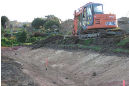
Fig.5 Excavation, preparation of side slopes to form channel
