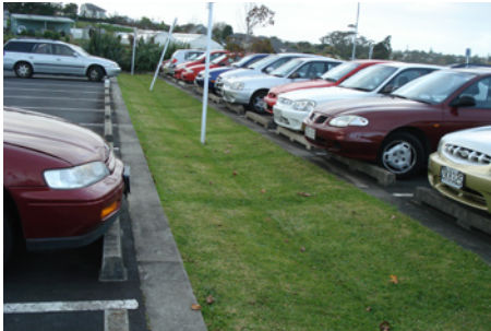
Fig.2 Waitakere City Hospital car park swale
