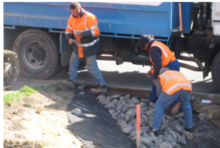
Fig.6 Construction of inlets with erosion protection
