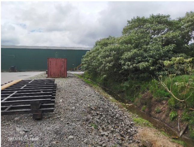
Photograph 3. View north along the western side of the bund showing existing drainage. Binstacker building in background.
