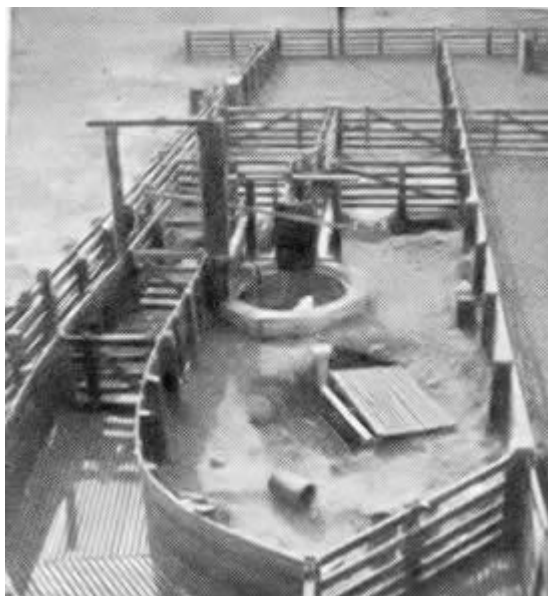
Photograph 11: Pot bath with curved race and covered sump http://www.mfe.govt.nz/publications/hazards-land/html/appendix-10-photographs-sheep-dip-structures
