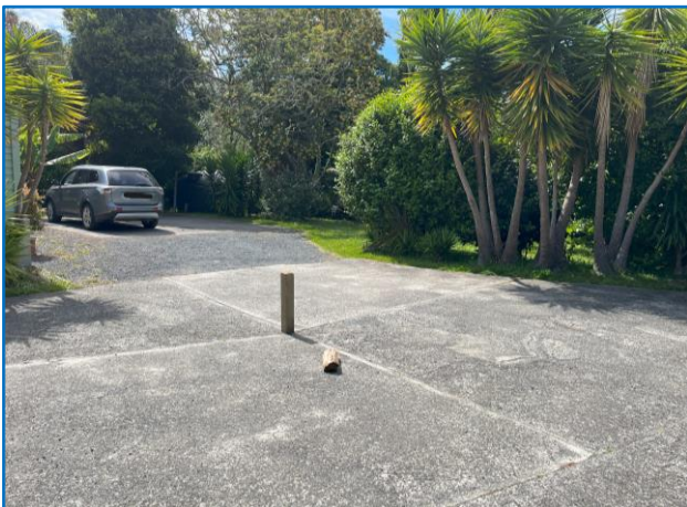
Photograph 3: Existing concrete parking area on Lot 2.
