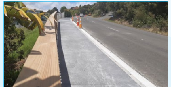
Cable Bay's new footpath includes kerbing and a wooden guard rail.
