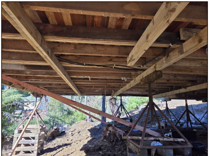
150 × 50 mm joists at 500 mm centres.
