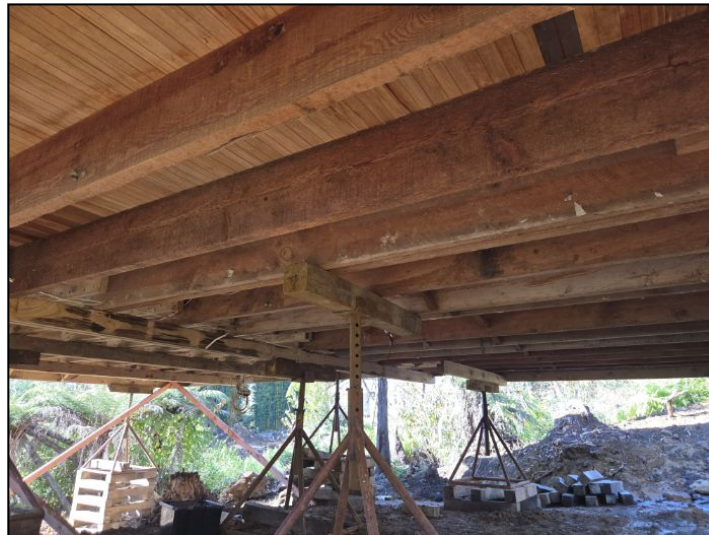
Oregon timber joists installed.
