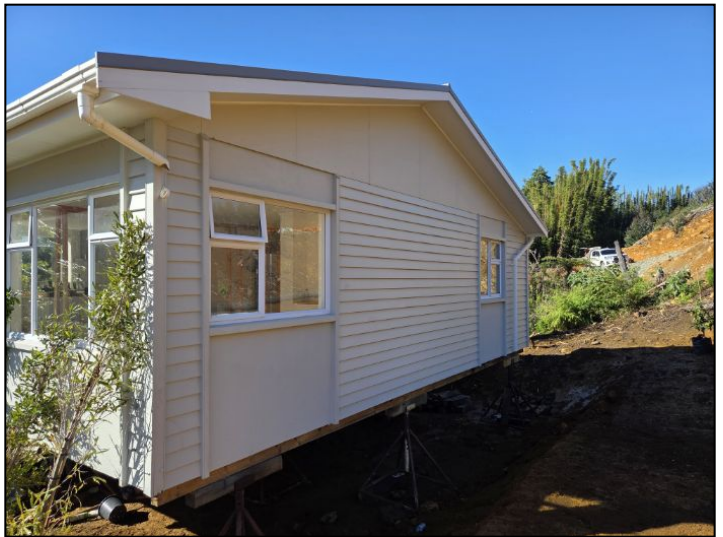
Painted timber weatherboards installed.
