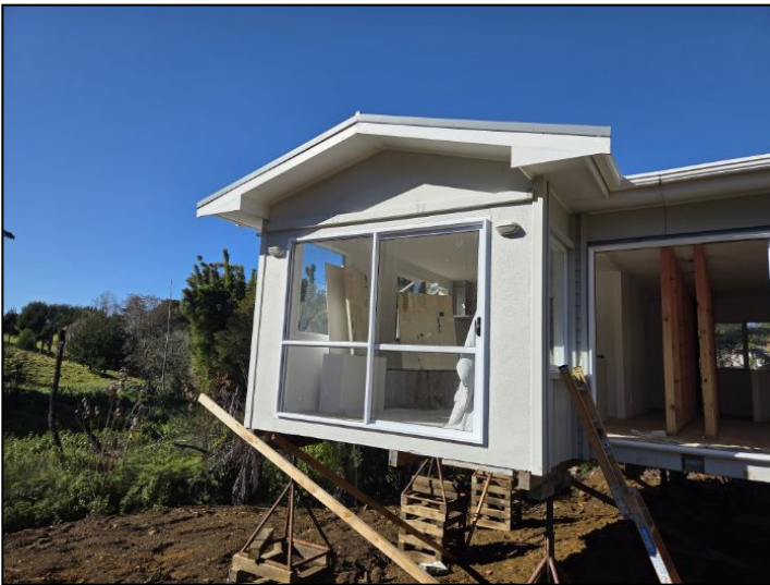
Textured Compressed sheet claddings installed.
