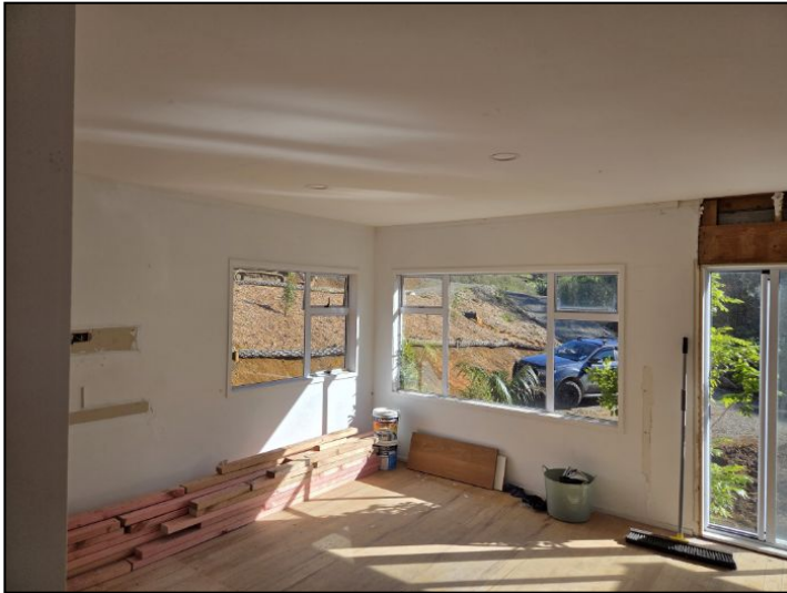
Gib plastered ceilings installed.
