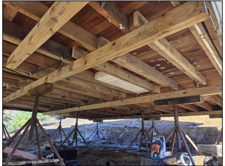
Rimu timber joists installed.
