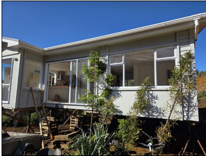
PVC gutters installed.
