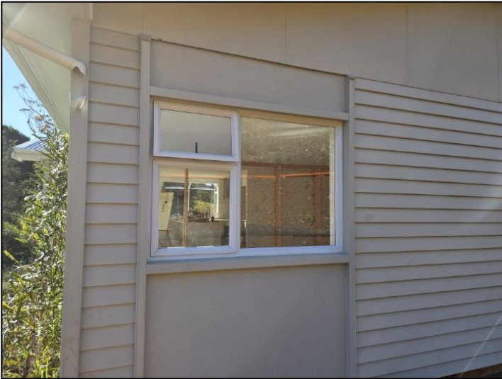
Aluminium joinery installed.
