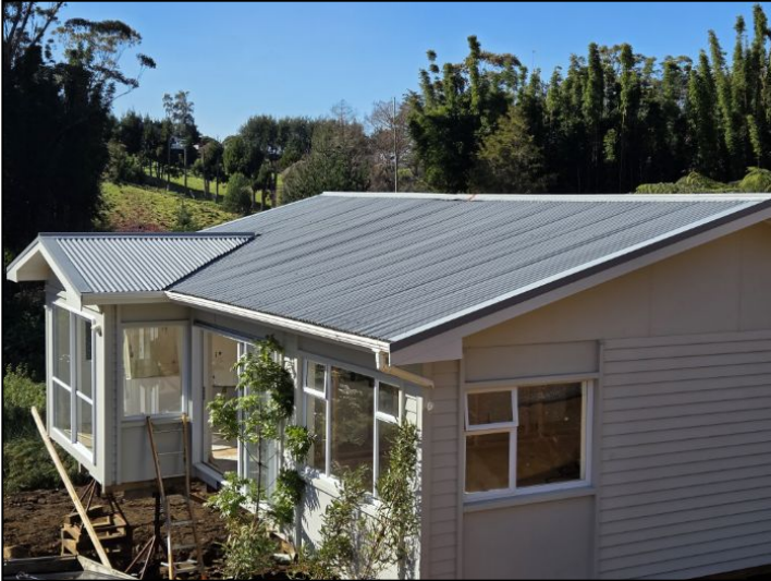
New zincalume roofing and flashings installed.
