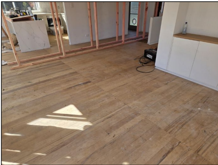
Timber T&G flooring installed.
