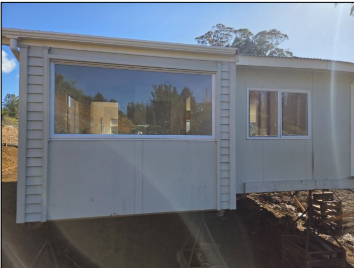
Timber fascias. Compressed sheet soffits and eaves.
