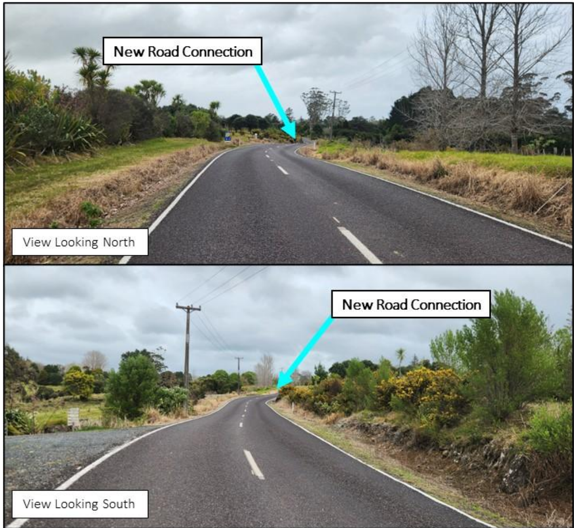
Figure 3: Proposed Road and Kerikeri Inlet Road Indicative Safe Intersection Sight Distance Image Source: Traffic Planning Consultants Ltd.
