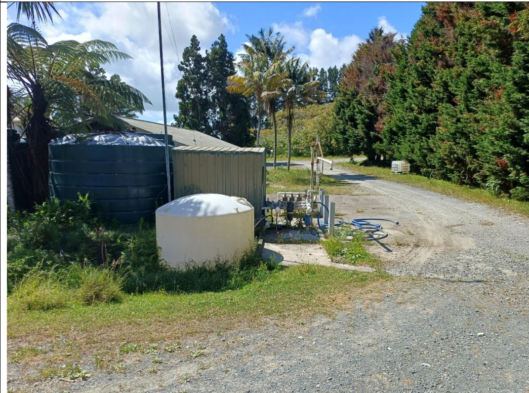
2. Irrigation point used for spray mixing, outside of piece of land.
