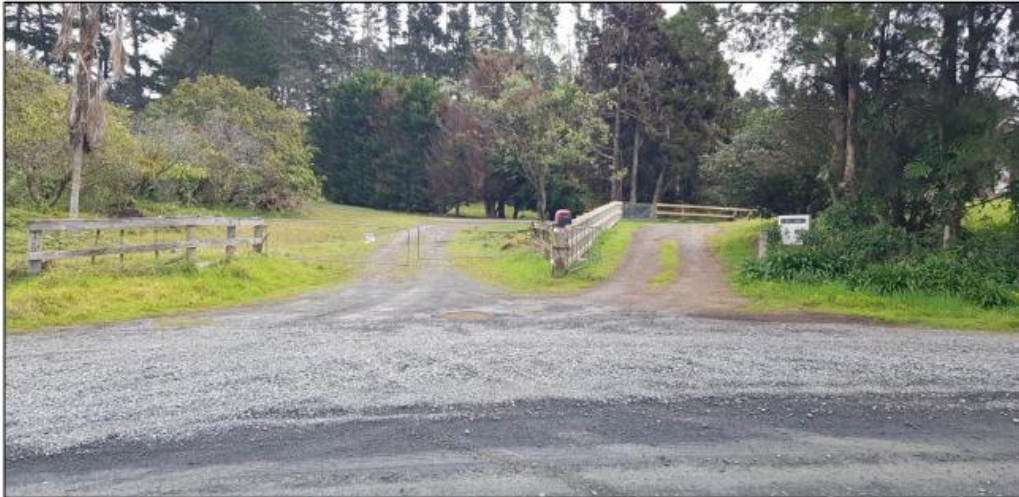
Figure 13 - Lot 5 existing crossings (left farm entrance, right house entrance)
