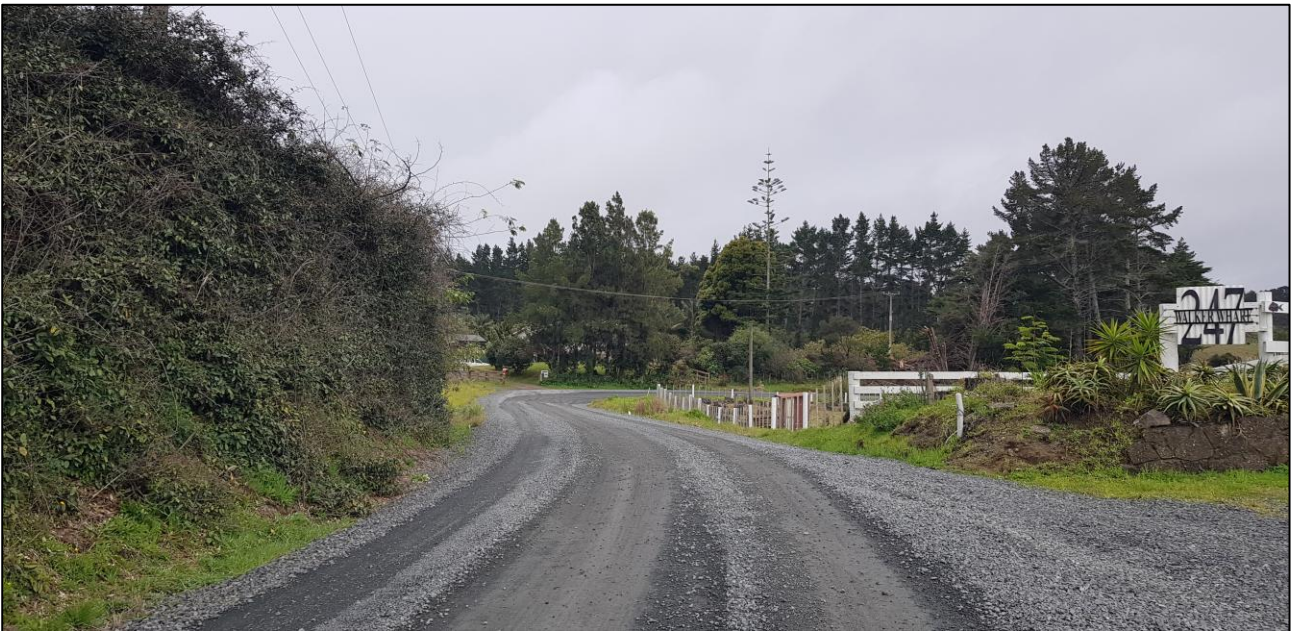
Figure 8 - Sweetwater Road north of Bird Road intersection looking north
