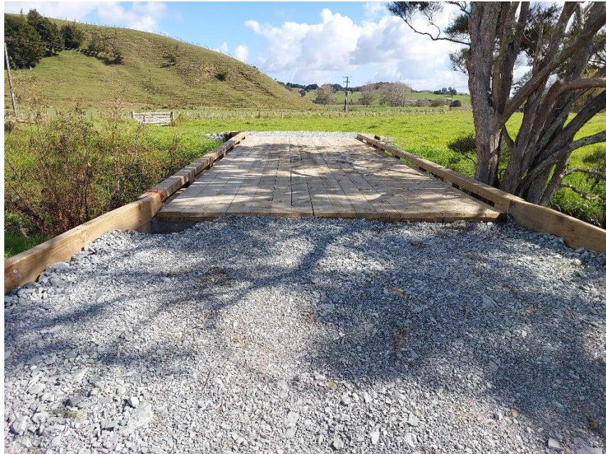
Newly constructed bridge looking back towards Orakau Road
