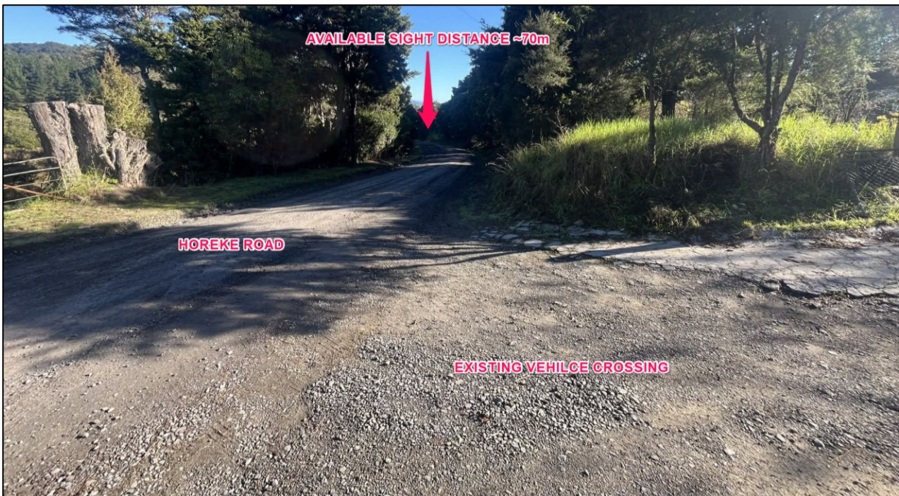
Figure 7: Annotated site photo from vehicle crossing show available sight distance to the north
