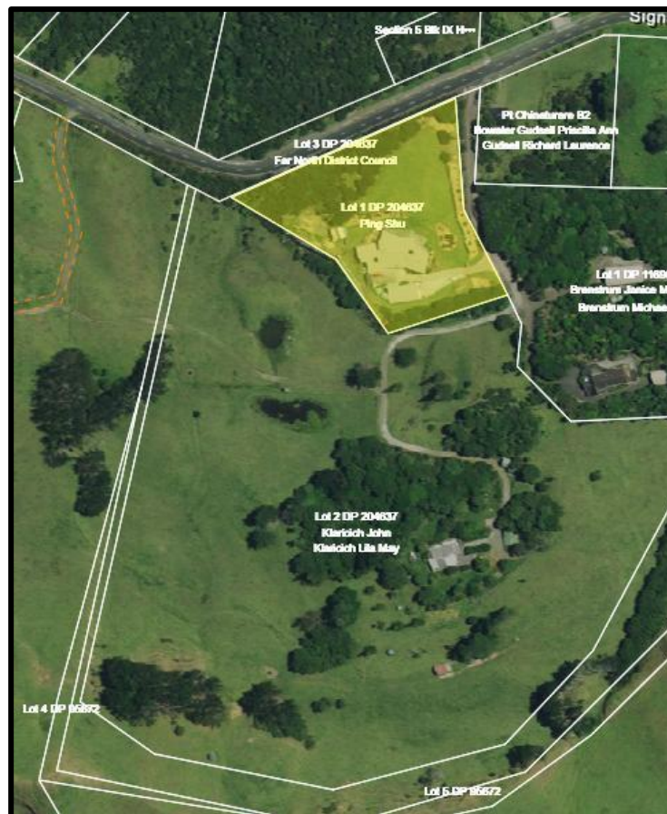
Figure 8: Image showing Lot 2 DP 204637 which adjoins the subject site and is subject to the setback infringement.
