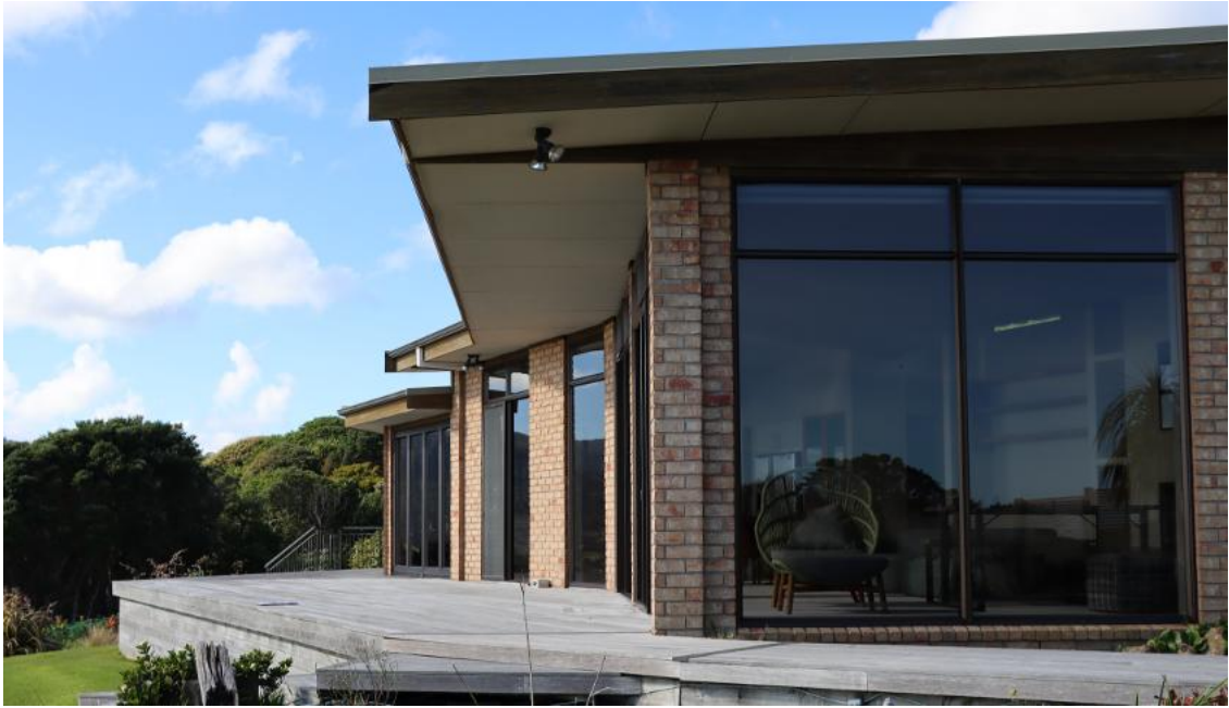
Figure 1: Existing dwelling exterior and glazing
