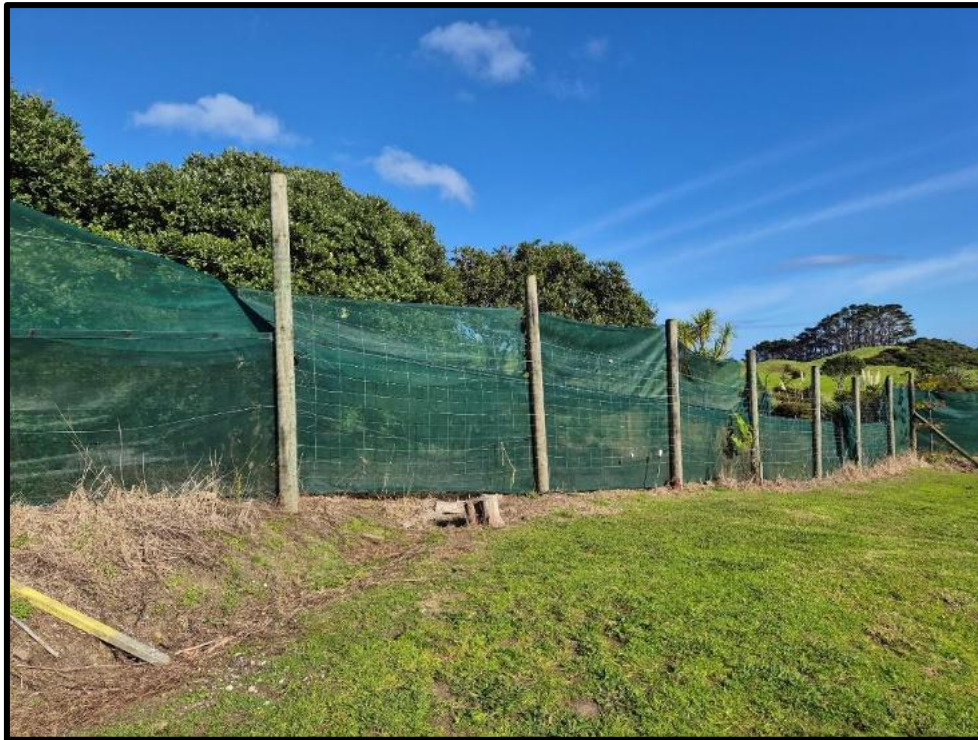
Figure 9: Existing meshing and poles which will be removed, along dividing boundary of subject site and Lot 2 DP 204637. Vegetation located on opposite side of fence is protected.
