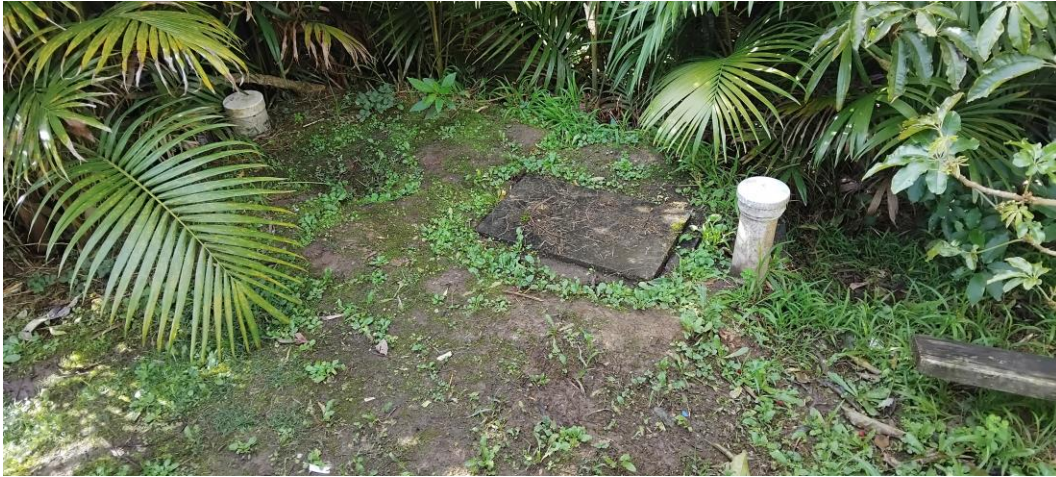
Figure 3. Existing buried septic tank (Lot 4)
