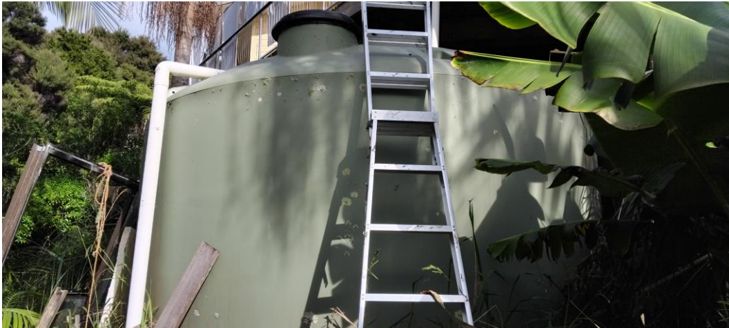
Figure 4. Existing water tank (Lot 4)
