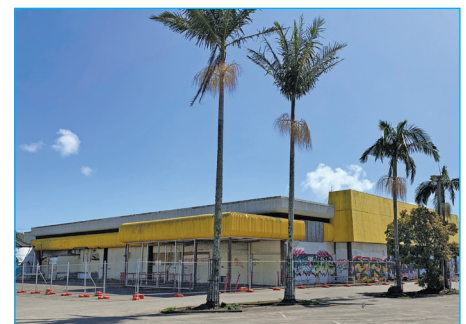
Works around the carpark will be carried out in conjunction with the Te Hiku Working Group as part of the Te Hiku Revitalisation Project.
