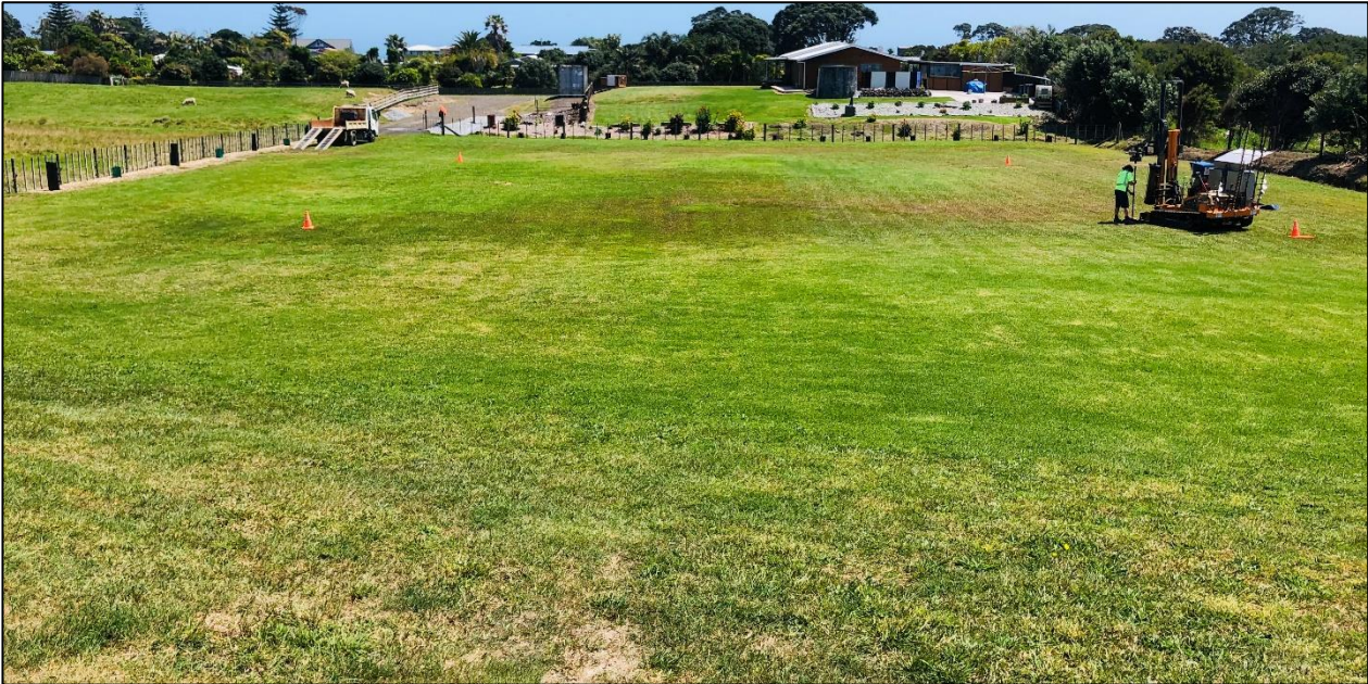
Figure 3: Site Photo – Overlooking the Nominated Building Platform in Lot 2. Orange Cones are Indicative of the 30m x 30m Investigated Platform.
