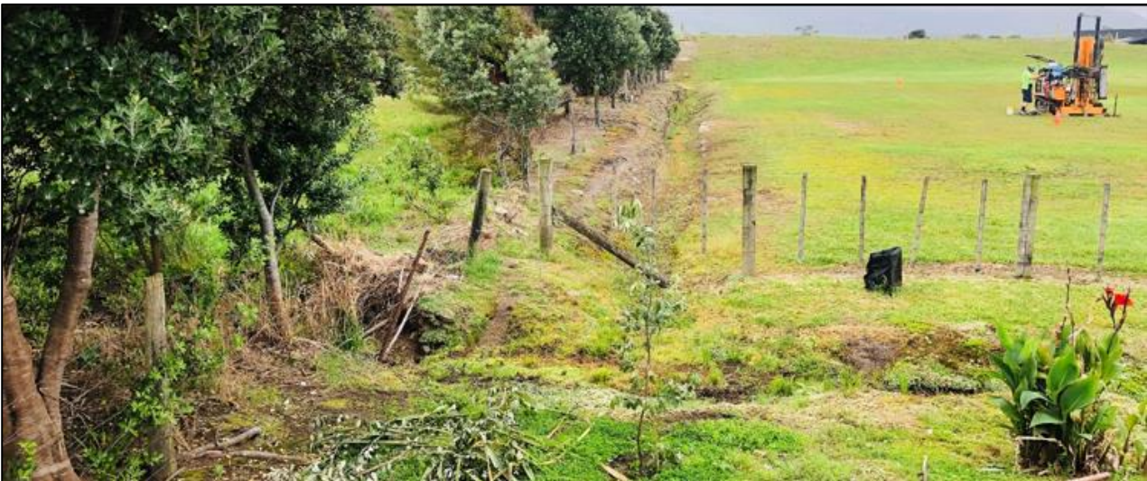
Figure 3: Site Photo – Overlooking Drainage System Along Northern Boundary to the left.
