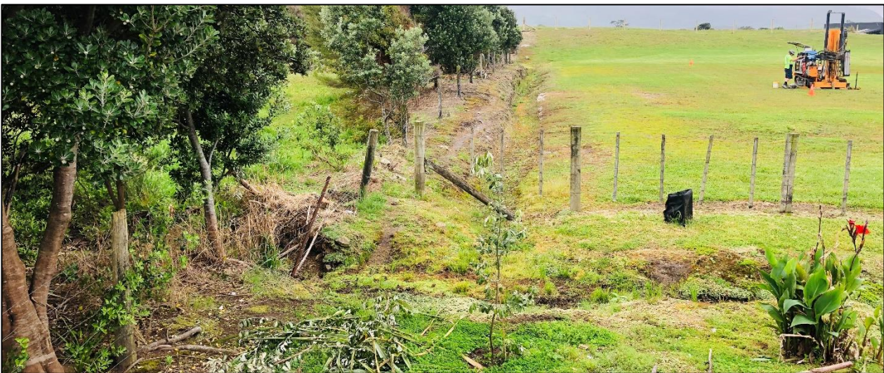
Figure 4: Site Photo – Overlooking Drainage System along Northern Boundary to the left.
