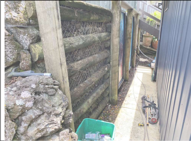
Photograph 3: Existing wall along northern side of house to be replaced with RW02.
