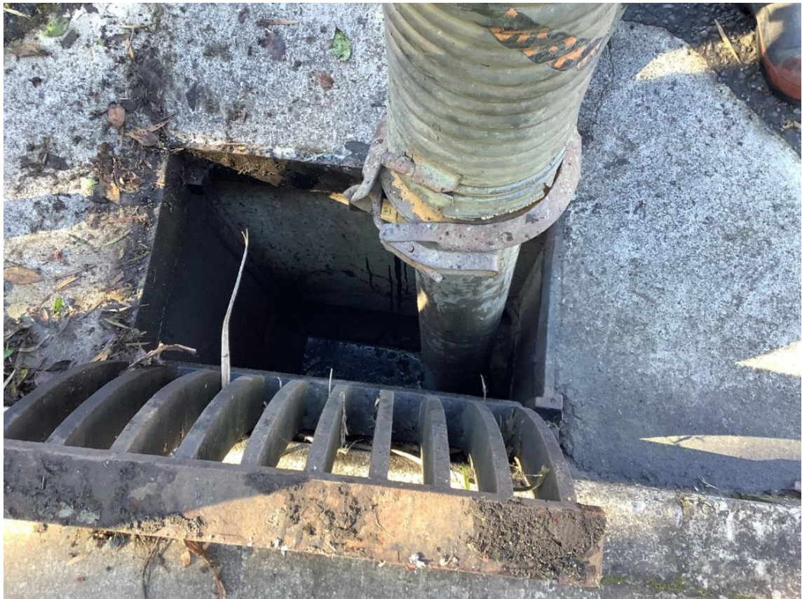
Bank St, Kaitia – Cesspit chamber clearing
