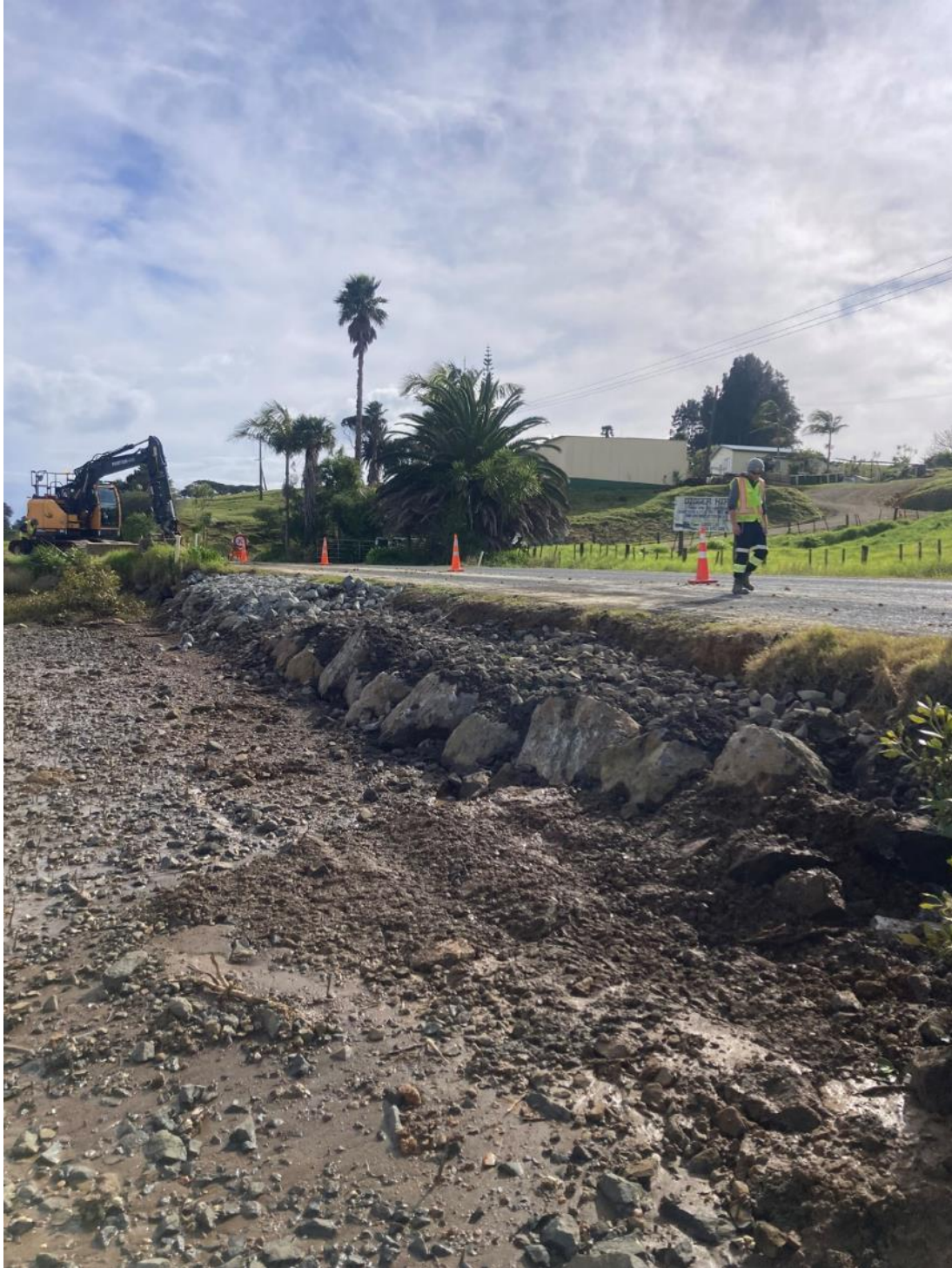
Hihi Rd – Rock Wall Repair in Progress
