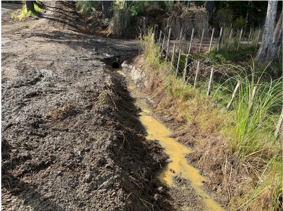
Yuretich Rd – Culvert End Clearing
