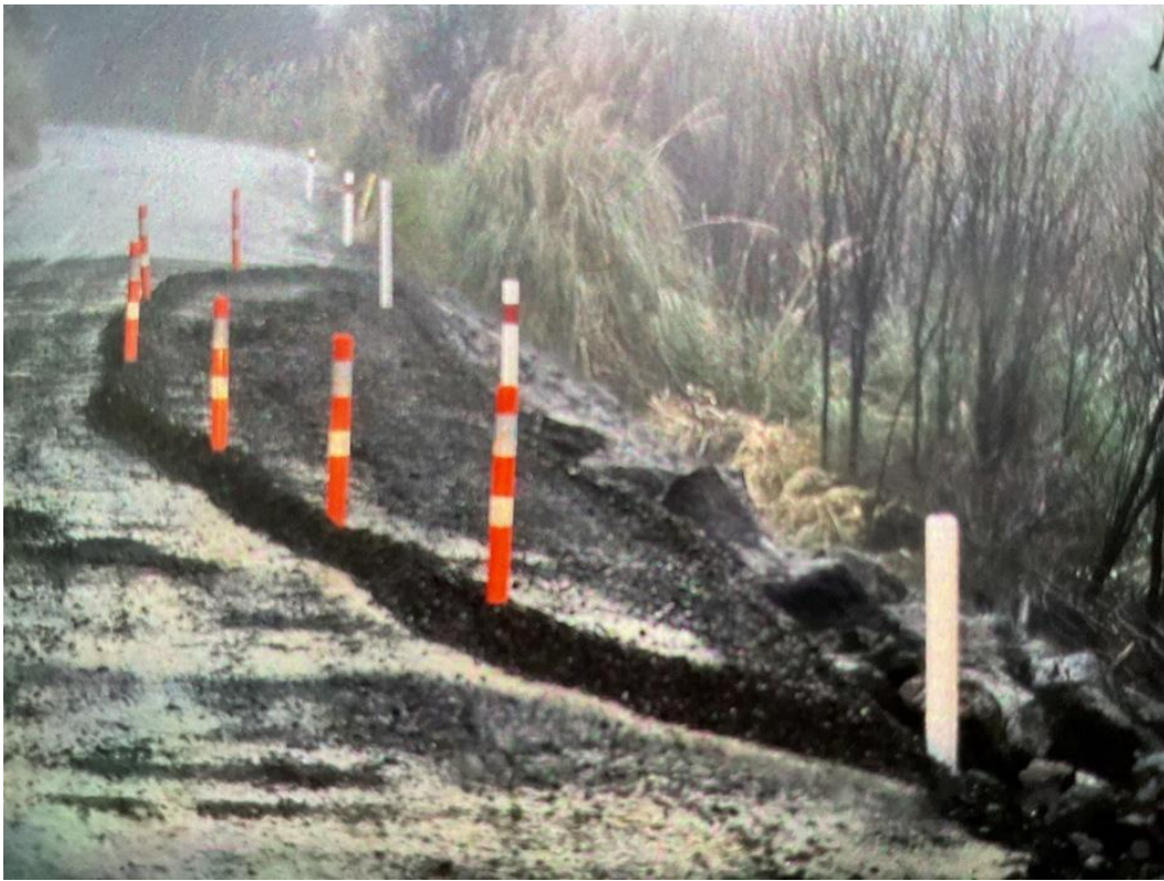
Paranui Rd – Bund and delineate Underslip
