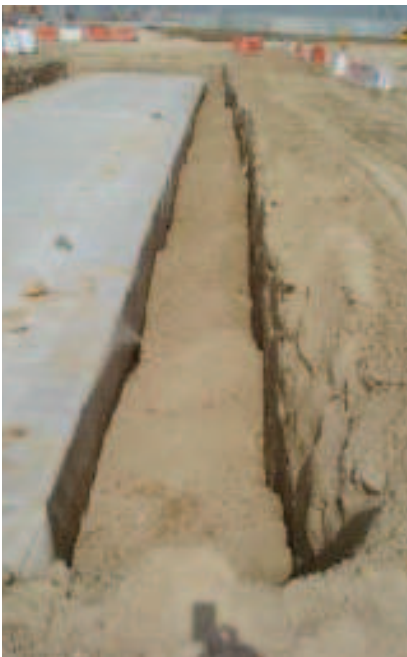
Fig. 22 Vibratory compaction of side backfill is always required , regardless of what backfill material is used.
