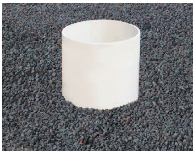
Fig. 17 Install port into RainSmart System
