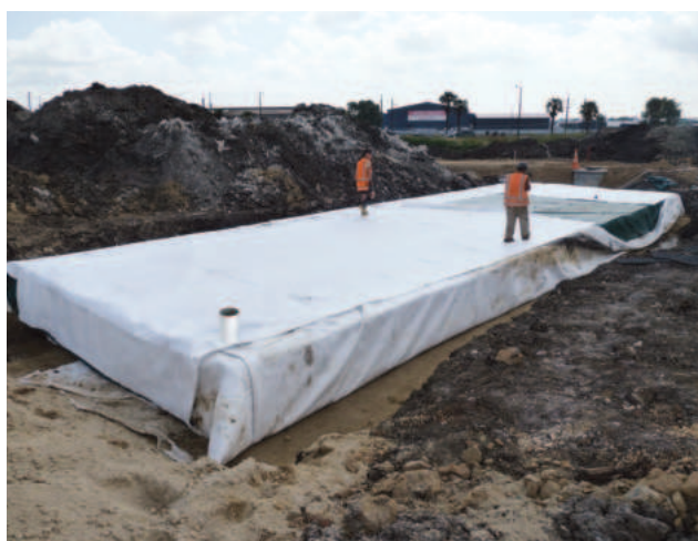
Fig. 16 Installed maintenance port
