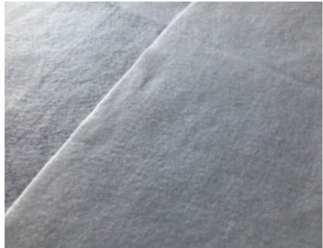
Fig. 7 Overlap geotextile by a minimum of 300mm
