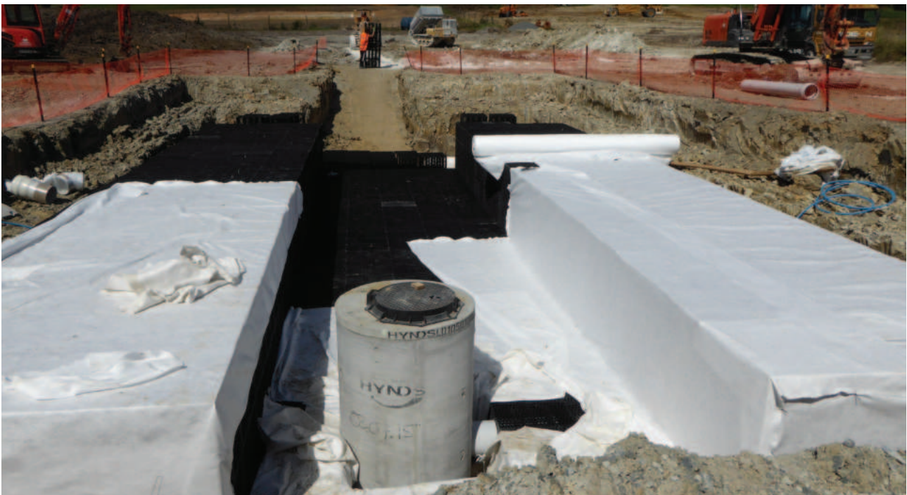
Fig. 18 Encapsulate RainSmart system with geotextile
