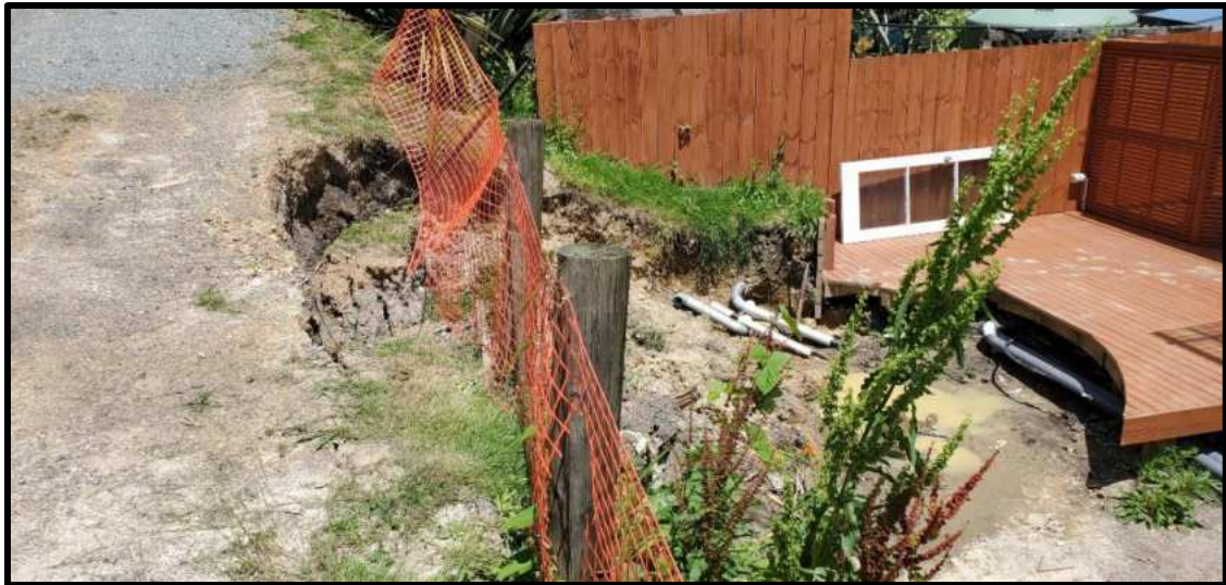
Figure 13: Image of slip from driveway along boundary with 21 Baker Street.
