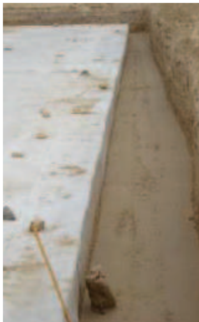
Fig. 22 Vibratory compaction of side backfill is always required , regardless of what backfill material is used.
