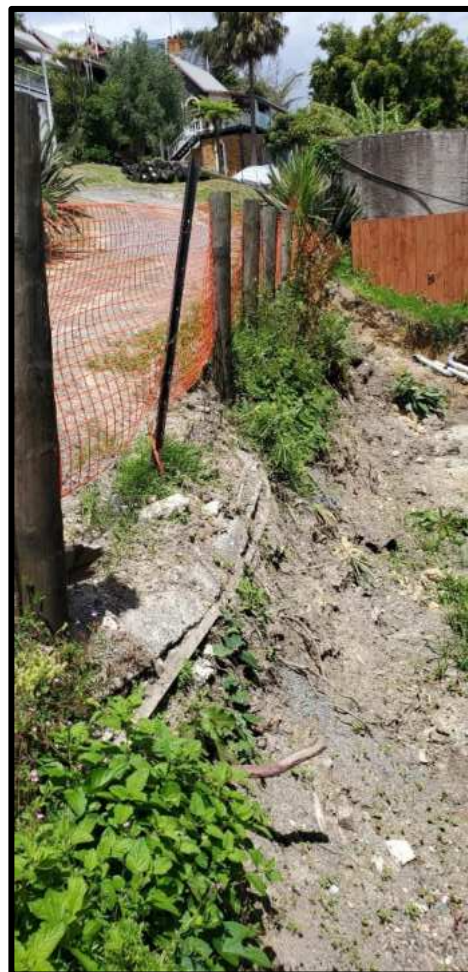
Figure 9: Existing slippage into 21 Baker Street.
